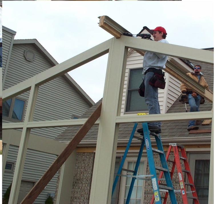
Before installing the first panel, install the C Fascia to the adjustable F at the ridge and fasten the C Fascia to the house at the overhang.
