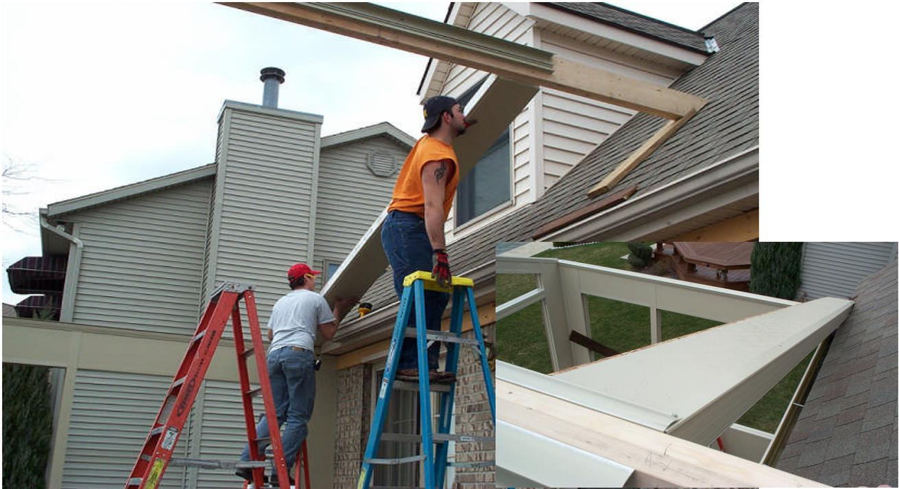
Rip the first panel so that the overhang on the front of the enclosure will come out even. Install the rest of the panels. In some cases it may be necessary to brace the side walls so they will not kick out & cause the beam to twist, this can happen when you try and put all the roof panels from one side then the other.
