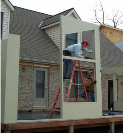
The walls can be laid out on the ground or stood in place to determine the roof pitch & notch for the beam. Chalk a line and cut the panels.
