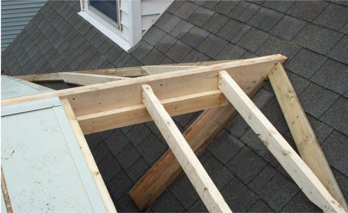
Make sure all the rafters are lowered  $7/16$ "s or  $1/2$ ", so the OSB will meet up flush with the Enclosure top.
