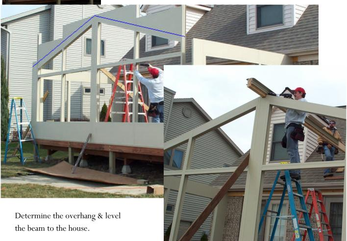
Before installing the first panel, install the C Fascia to the adjustable F at the ridge and fasten the C Fascia to the house at the overhang.
