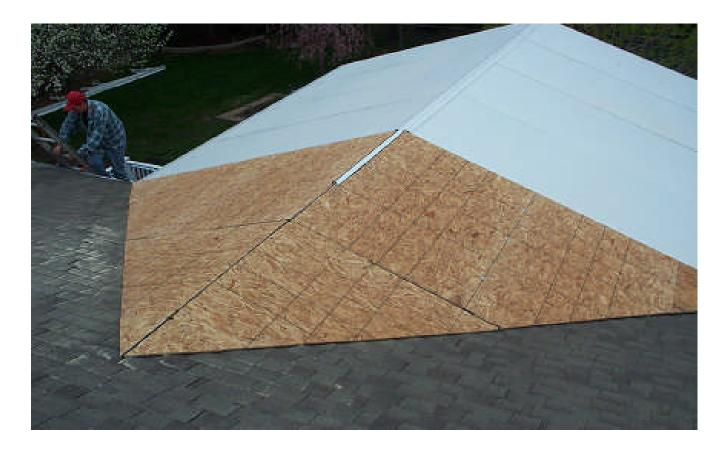
Chalk a line and cut the existing house shingles clear down below the tar paper. Install "Ice Shield" or valley flashing, 5 to 6 inches up under the existing house shingles.
