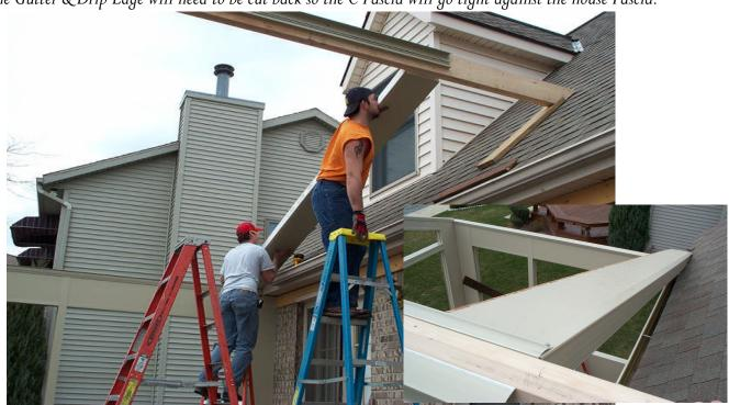
Rip the first panel so that the overhang on the front of the enclosure will come out even. Install the rest of the panels. In some cases it maybe necessary to brace the side walls so they will not kick out & cause the beam to twist, this can happen when you try and put all the
