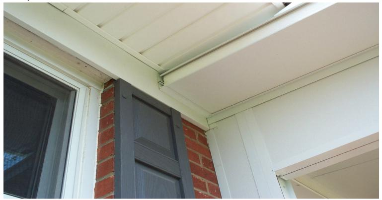
Start snapping the rest of the panels into place.
