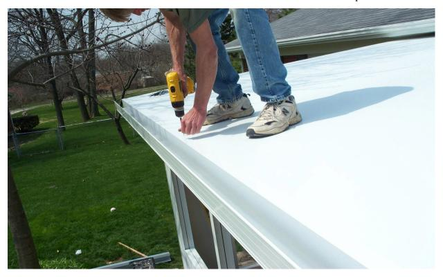
Measure the C Fascia from the house to the front of the G Fasica, notch the C around the G.
