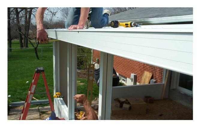
Lag the roof panel down so that it pulls the F Channel below up tight against the roof panel.
