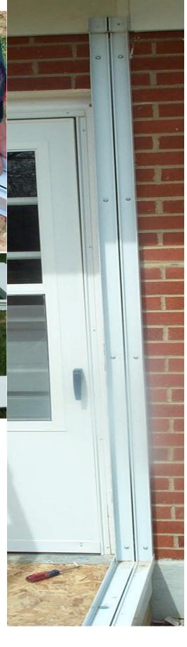
After the wall has been cut down to size, start inserting the wall panels.
