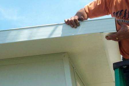
Corners can be mounted to the inside of the F Channel at the bottom and outside at the top.
