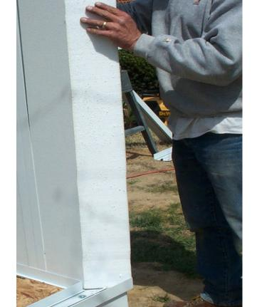
The corner spline installation, will be the last wall panel to install, they have already been mitered.
