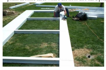
the highest measurement & work to the lowest. **Note:** Wall panels may be cut with a 7 1/4" circular saw with a plywood blade.
