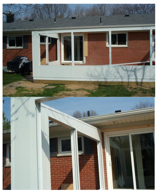
Secure the Vertical Wall Channel with 1/2" hex head tec screws.
