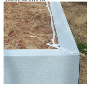
**Note:** If wall is being installed in a confined area, it may be necessary to rip the F Channel. If this is the case, secure the wider section to the floor sides & roof.
