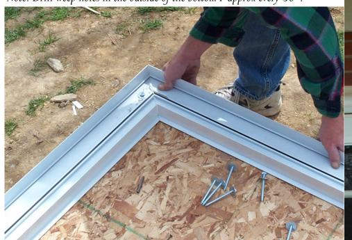
Caulk the back of the U Channel to the house wall and fasten with concrete anchors, this is the starting point for the walls.
