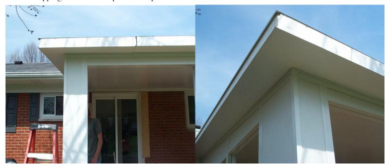
Secure the roof panel to the wall below with the 5" lags, measure in from the front edge of the wall, making sure it's plumb.
