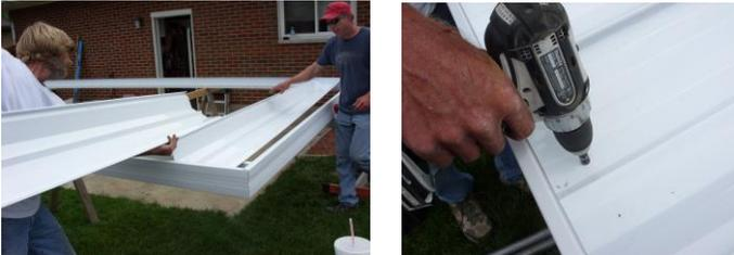
10) Install front corner angle. Caulk and secure with (2) screws on each side.
