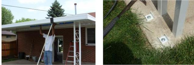
8) Install awning pan with the box end (female) against fascia, this allows for easy locking of additional pans. Slide the pans to the rear so the pre-punched holes line up with the lower lip of the fascia. Secure first pan to side fascia top lip with hex head screws, approximately 12". (Last pan will be secure in same way)
