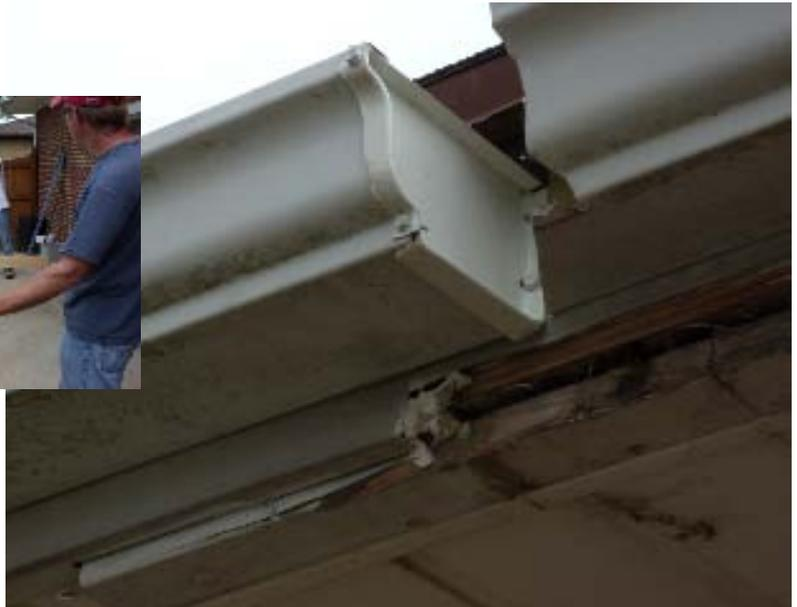
Cut the existing house gutter and cap each end with a left and right gutter cap. then mark the rafter tails, or studs ( for wall mount)
