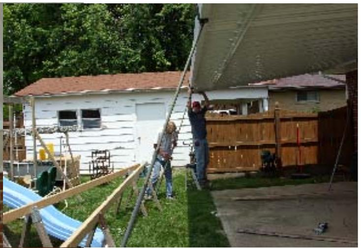
Lag awning thru your predrilled holes for each rafter tail.
