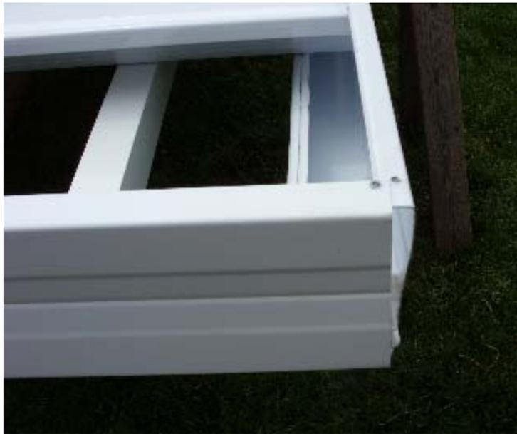
Push corners back together and reinstall the screws. Screw the side "C" Fascia in the top lip down into the pan approx every 1 1/2 feet.
