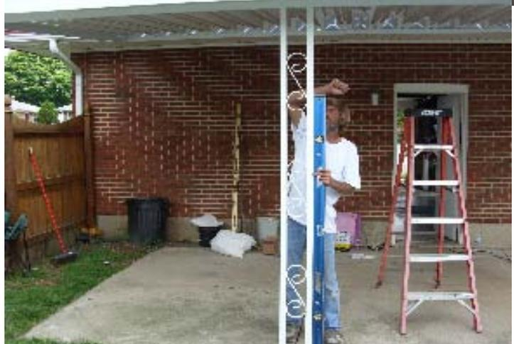
Plumb the posts and mark around the foot of the posts, set post back off of you mark and set the post foot in place to mark where the hole will be drilled.
