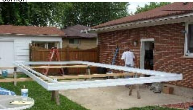
Scribe pencil mark in groove of gutter to help see thru pan holes for when they get screwed on later.
