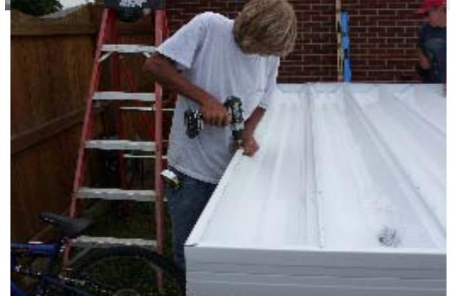
Caulk the inside of each of the 4 corners and attach them to the frame using 4 screws on each.
