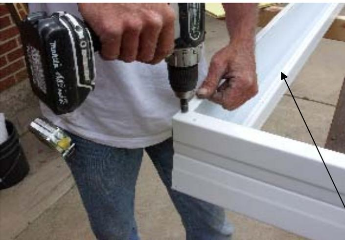
Install a 1/2" Tec Screw in the top and bottom of the of each corner.
