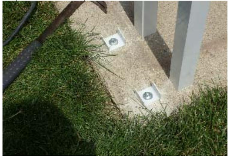
Lift post onto the post feet and fasten with 1/2" Tecs
