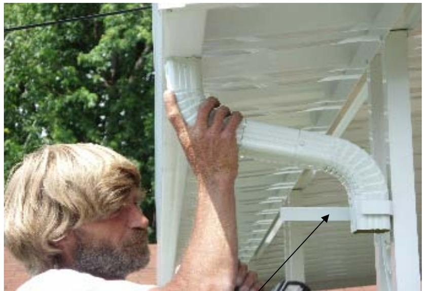
Fasten one gutter strap to the post toward the top of the D/S and the other strap toward the bottom as shown
