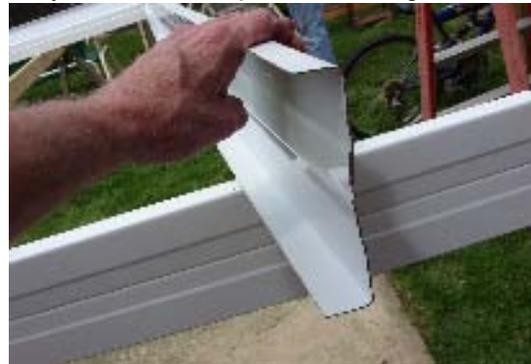
Assemble the frame which consist of the G and C Fascias
