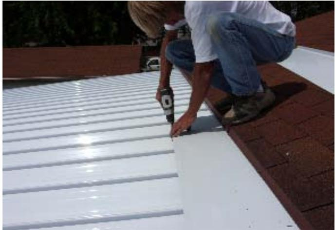
Scew down to each raised seam of the W-Pan and caulk all screw heads.
