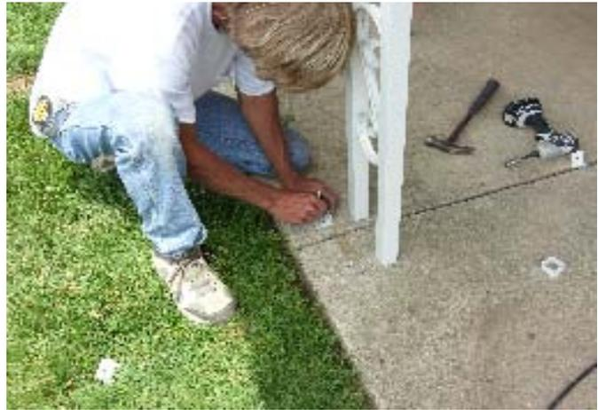
Drill a 3/8" hole into the slab with a concrete bit and mount the post feet with an expansion bolt.
