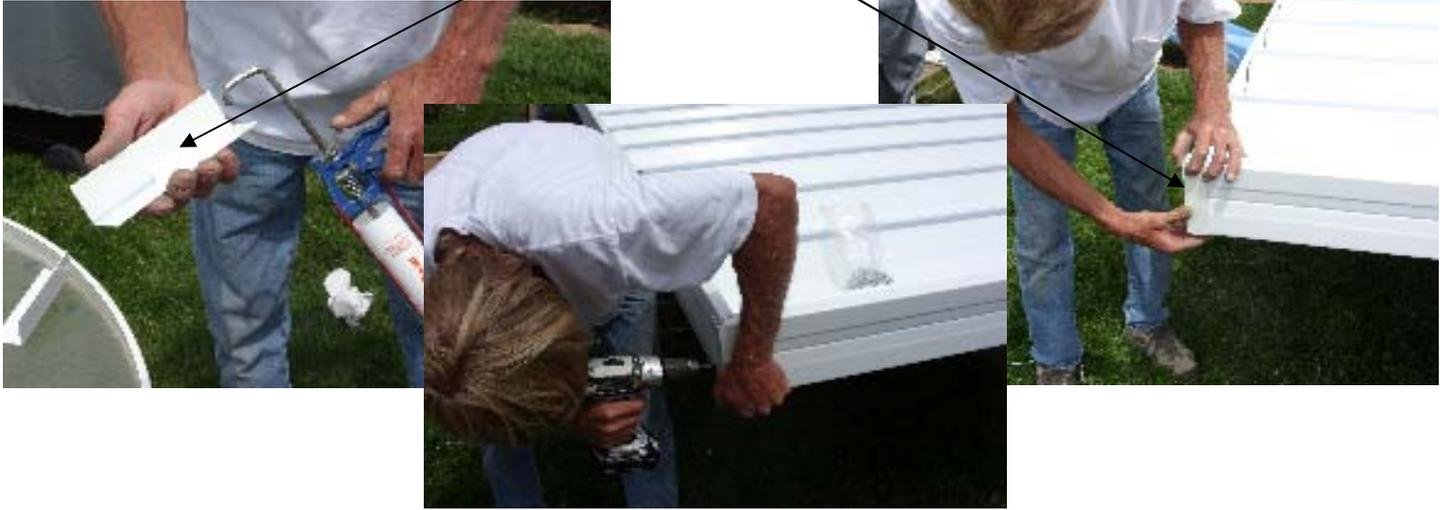
Locate exact position of the support and where it needs to be in relation to the concrete slab, screw the beam into place.
