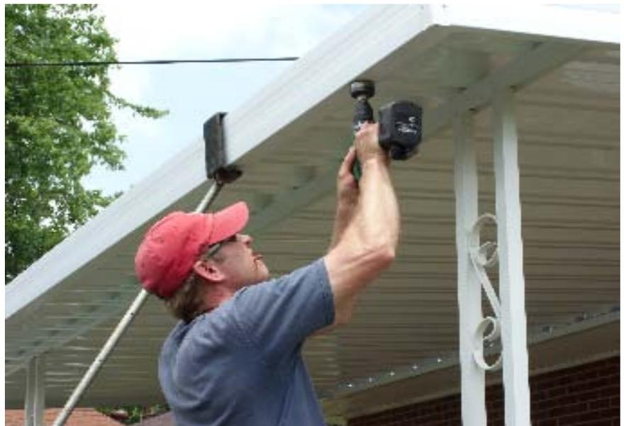
Drill 2 1/8" Hole into the bottom of "G" Fascia or Gutter
