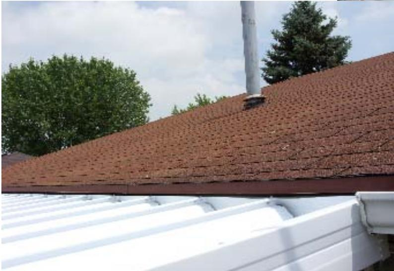
Adjust for the proper slope NO LESS THAN 3/4"
