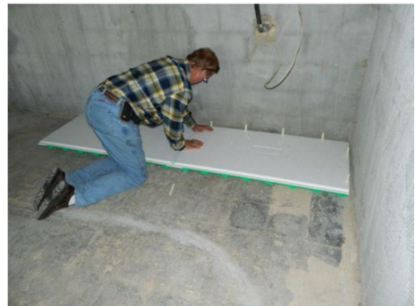
(Photo: James Wright) Skip Bennet installs the high-density foam panels that will help create a thermal mass slab.
