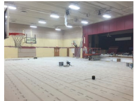
▲ It took nearly a day to put shell paper on the floor before prepping could begin.
