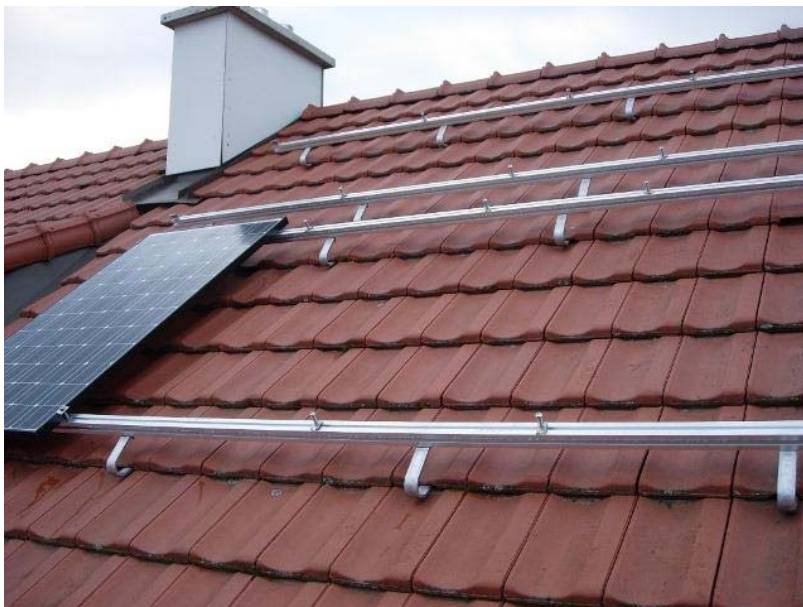
Photo 12: A tile roof hook mount bracket system
