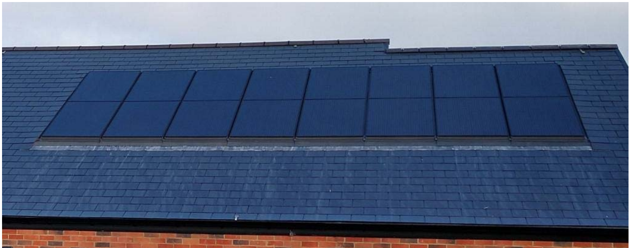
Photo 5: Integrated black PV panels
