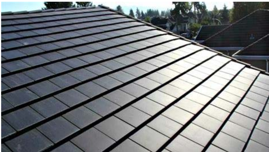
Photo 10: Tesla solar roof tile
