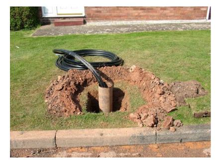
Photo 4: Pipework loop installed within a borehole
