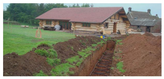
Photo 2: Horizontal ground loop (courtesy of CA Heat Pumps Ltd)
