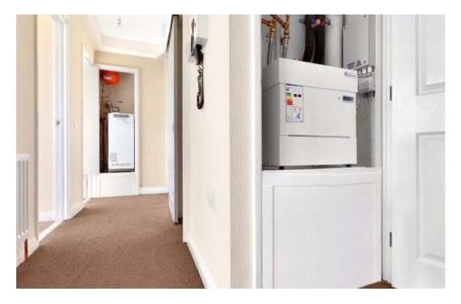
Photo 7: A Kensa 3kW 'shoe box' heat pump (photo courtesy of Kensa Contracting)
