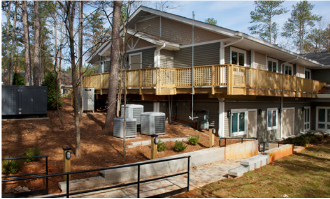
Full backup power by 175 kW generator
