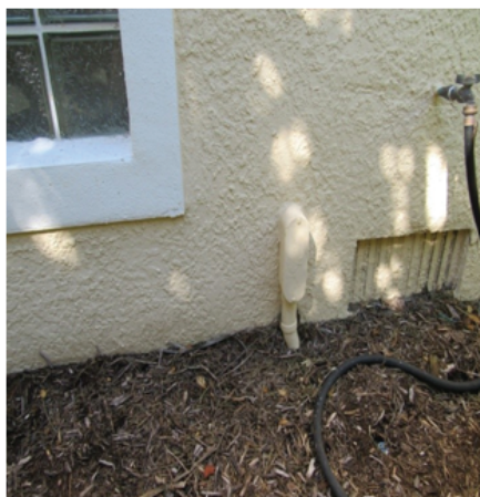
Picture 3: After 8 years of exposure to high humidity and hot air temperatures in the shade, no algae or mold growth appears on the surface.
