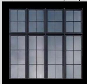
Adding grids is called a "simulated divided lite" that emulates windows with a more traditional look when they were made with smaller panes of glass inserted into the wood frame grid. The thin aluminum frames provide a more contemporary version of this timeless look.
