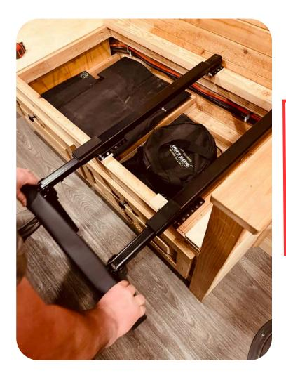
Step 10. After the rails are fastened down, verify that the rails slide freely in and out. If it is not straight, level and square; it may bind. Make adjustments if necessary to make sure it moves freely.
