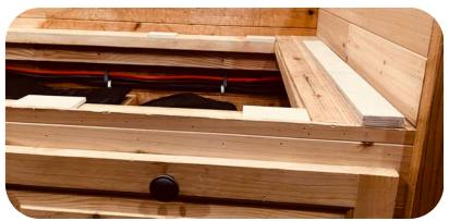
**Step 7.** Place your small wooden shims where you chose to mount the leg rest rails to assure the leg rest will sit level. Some places may not need a shim.
