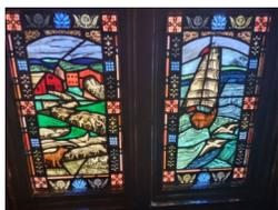
Apostles Window: The glazing compound around the exterior of the stained glass is dried out and breaking away from the window. There is a slight bow at the bottom of the window. The panel with the bowing will be removed and repaired. The exterior glazing compound will be removed and all stained
