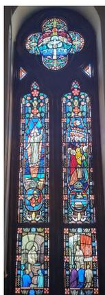
Ascension & Pentecost Window: There is bowing in the robe area of the right lancet. This window will be removed and completely restored. Once restored the window will be re-installed and new laminated glass protection will be installed on the exterior. Prior to the installation of the protection glass, the exterior part of the window frame will be scraped, primed, and painted.
