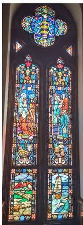
Epiphany & Presentation Window: There is bowing along the border on both sides of window running from the bottom to the top. This window will be removed and completely restored. Once restored the window will be re-installed and new laminated glass protection will be installed on the exterior. Prior to the installation of the protection glass, the exterior part of the window frame will be scraped, primed, and painted.
