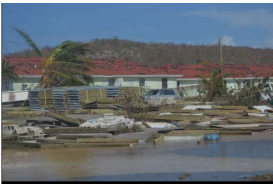
Figure 5: Petty's behind the main apartment complex flooded days after the hurricane passed.
