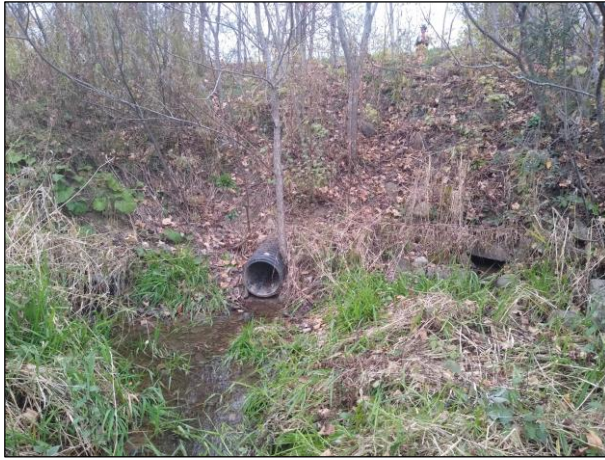
Photo 47: Outlet of three parallel pipes connecting Reaches FCT-3B and FCT-3C to downstream pond
