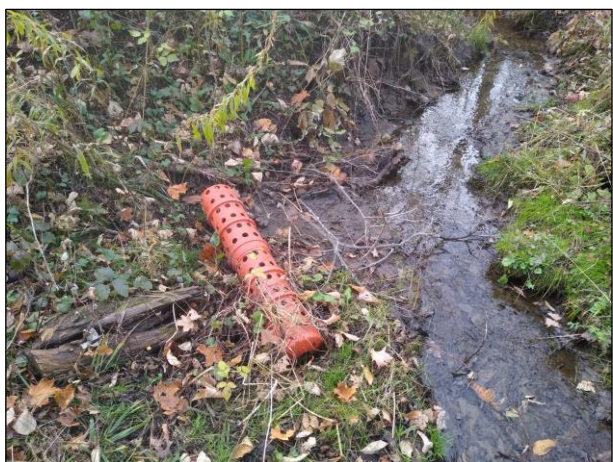
Photo 23: Fallen riser pipe
