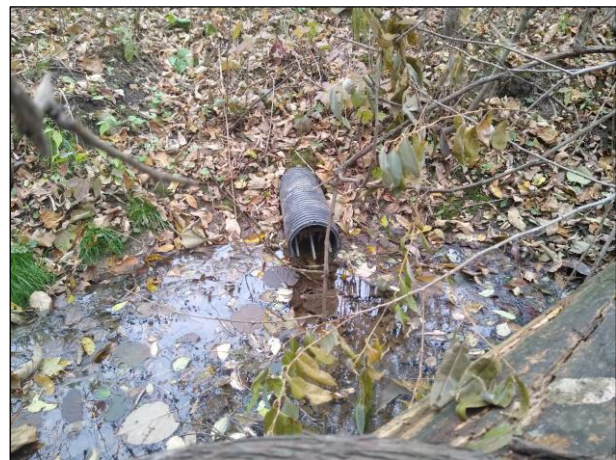
Photo 39: Tile drain outlet
