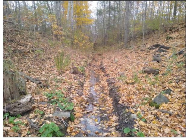
Photo 44: Excavated low-flow channel with exposed banks
