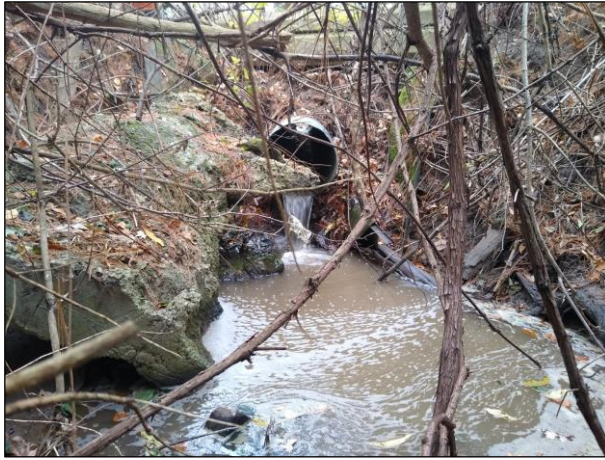
Photo 33: Perched culvert and plunge pool (facing upstream)
