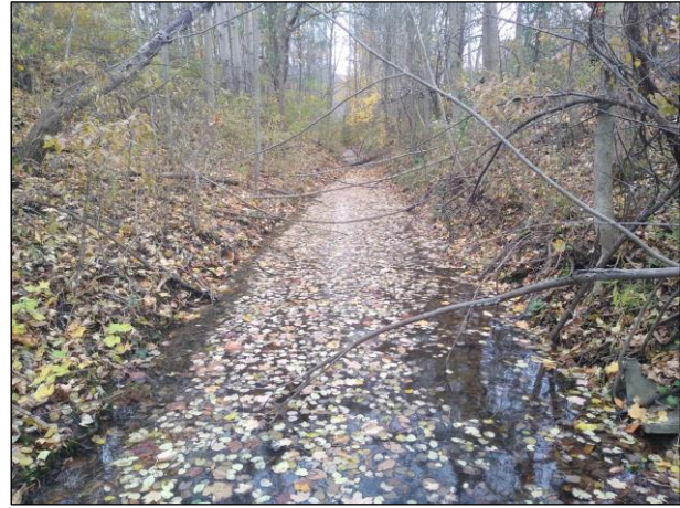
Photo 41: Straightened channel with localized erosion on right bank
