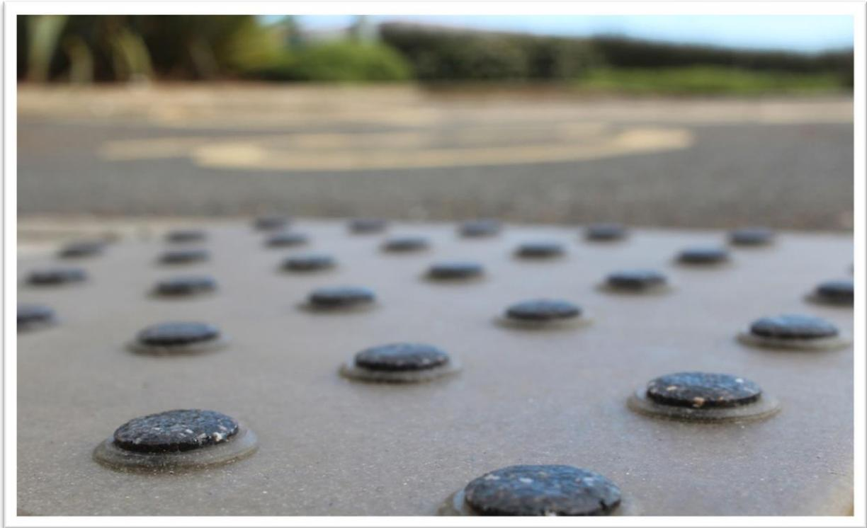
The tops of the blisters contain a diamond hard aggregate which is designed to contrast in colour to the rest of the tactile surface. As pedestrian footfall gradually wears away the tops of the blister a change of colour occurs that indicates the surface requires remedial maintenance.
