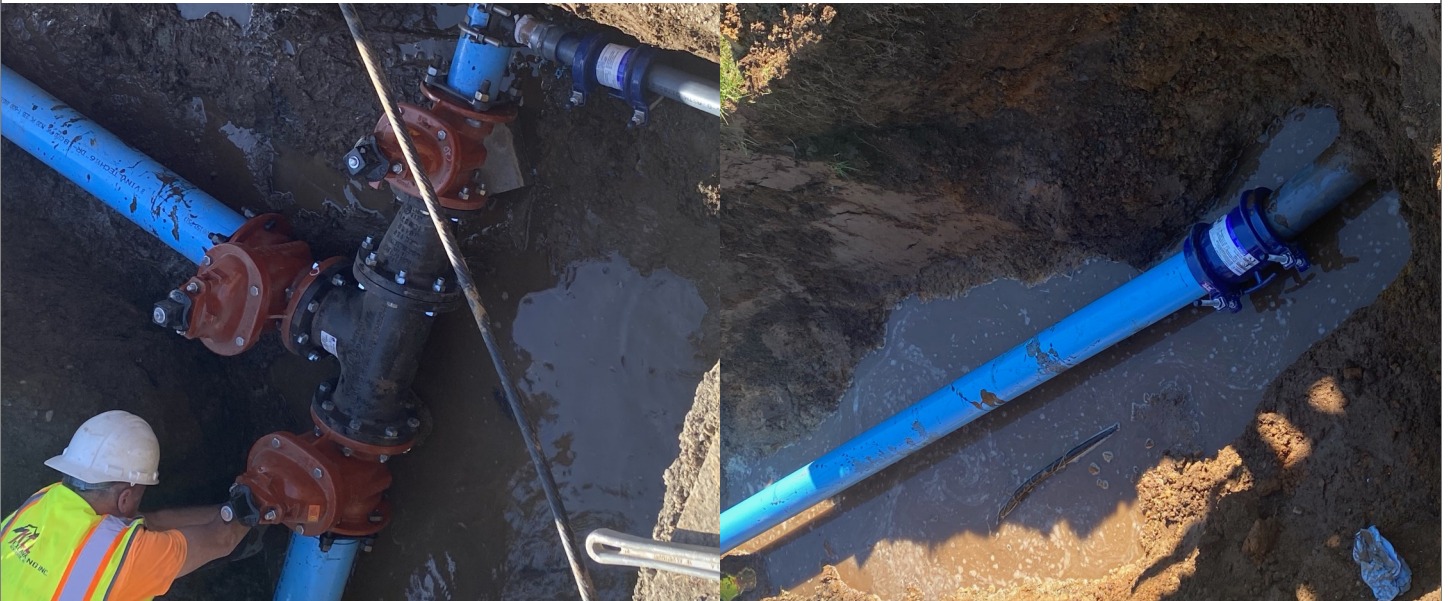
PICTURES FROM THE PIPE REPLACEMENT AT THE DAM
