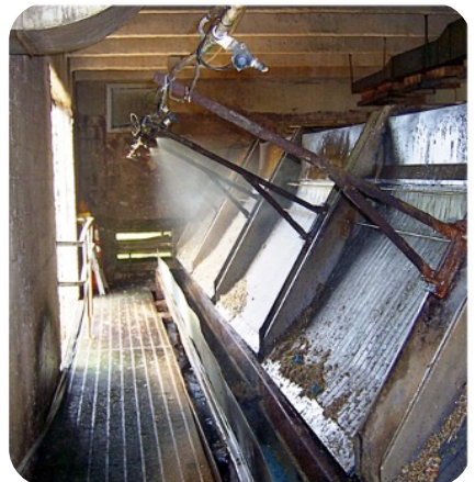
Synchronized misting system was installed at the screening station.
