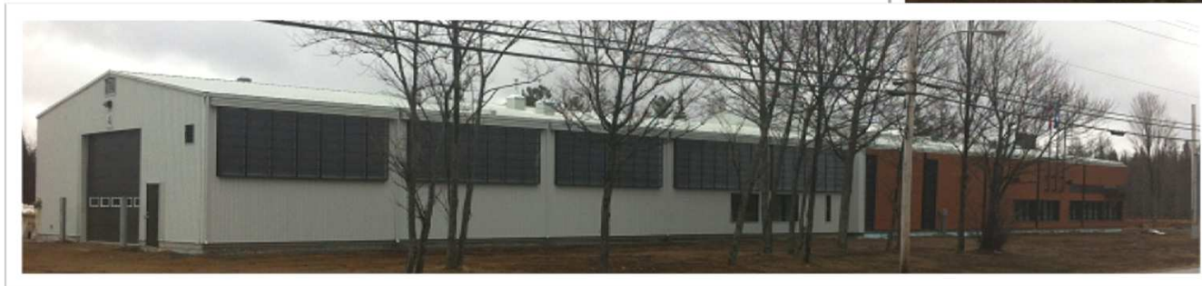
Garage municipal – Municipal garage – 74 m 2
