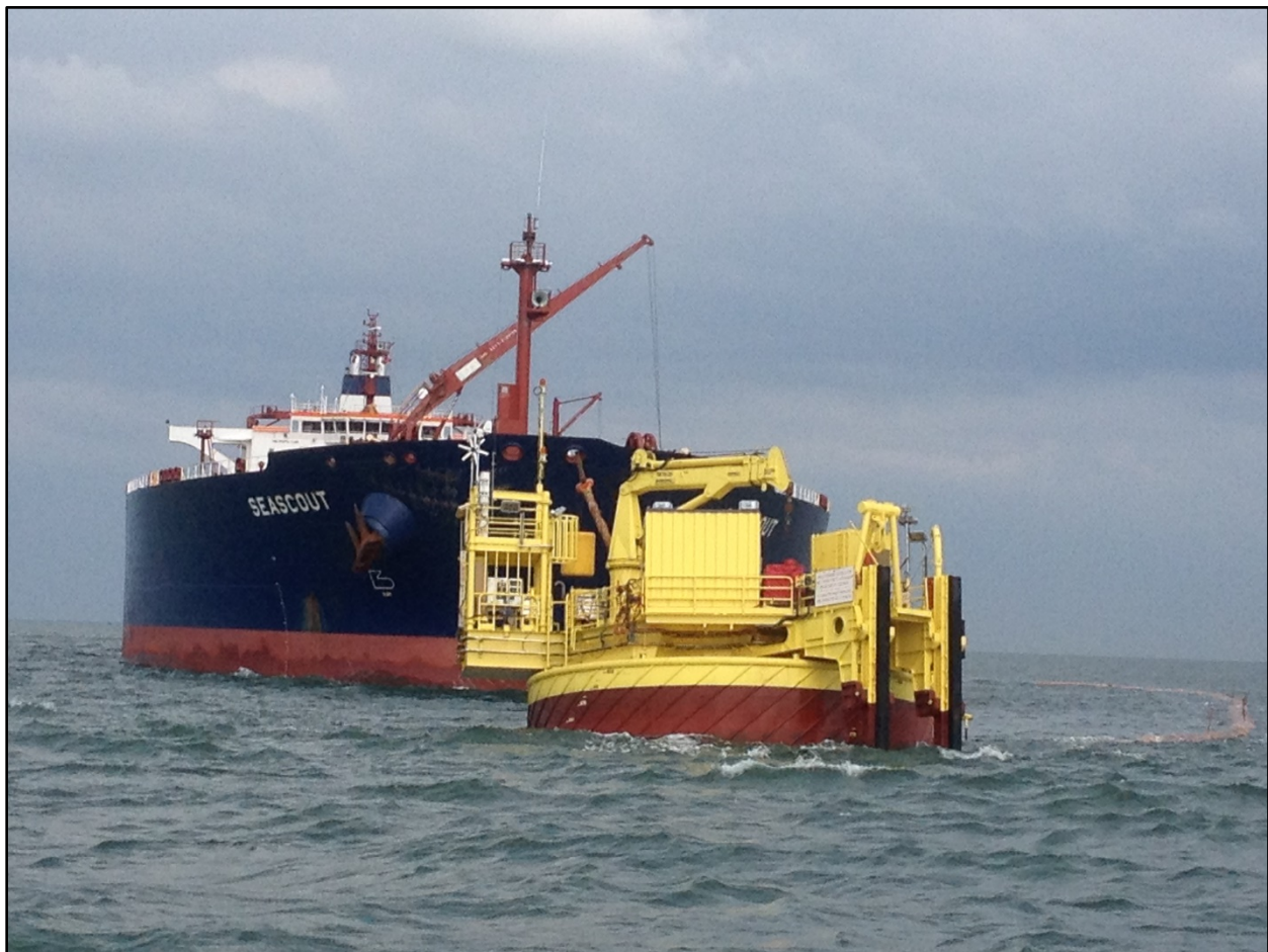
Figure 2-23: Single Point Mooring Buoy System in Operation
