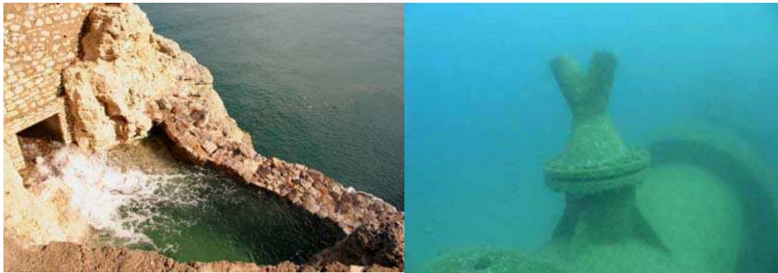
Fig. 3. Photographs of brine discharge configurations located in Spain. .A) Discharge trough a submerged outfall. B) Surface discharge .C) Discharge trough multiple jets (CEDEX).
