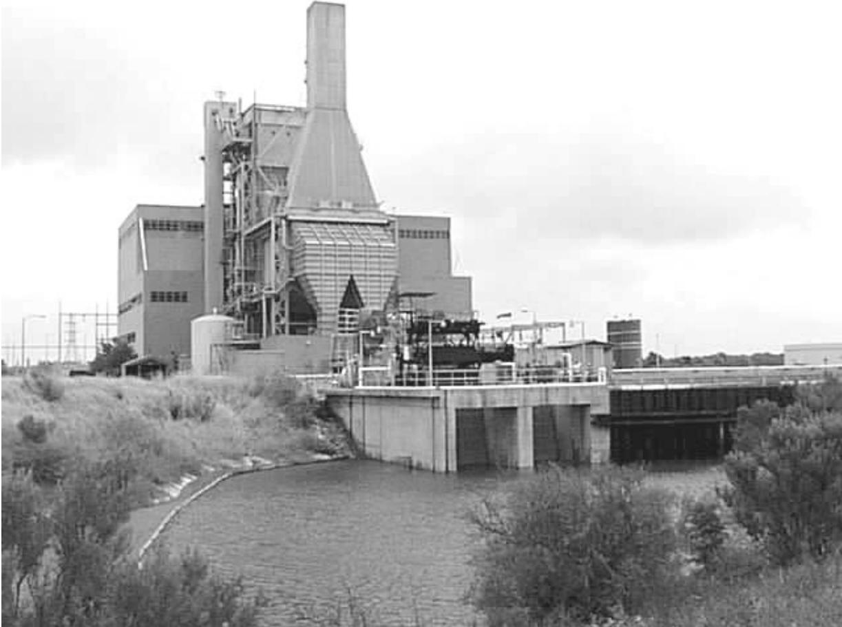
Figure 1 Typical surface water intake
