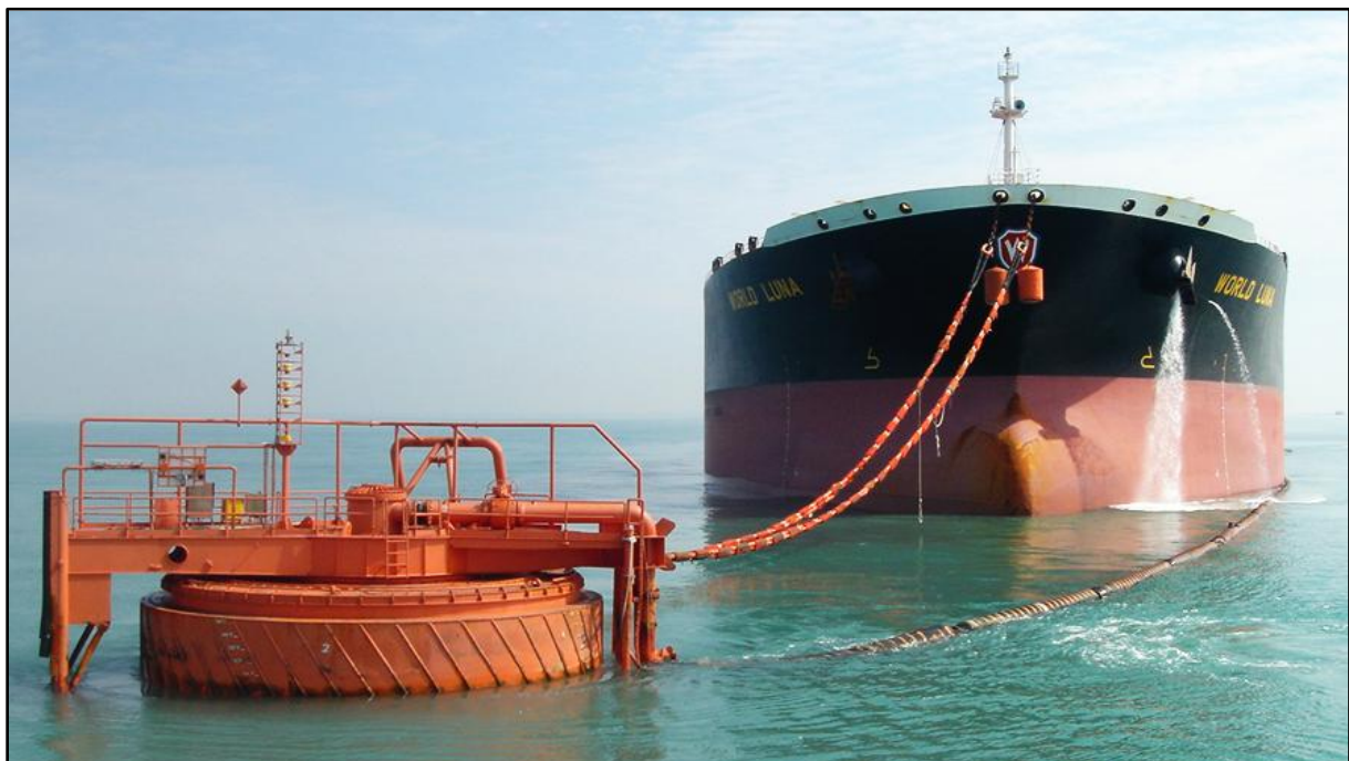
Figure 2-14: Single Point Mooring Buoy System in Operation
