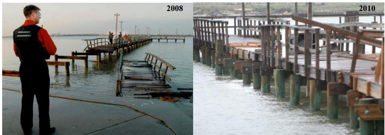
Figure 2. Examples of ship wave damage to fishing pier in 2008 (left) and 2010 (right).
