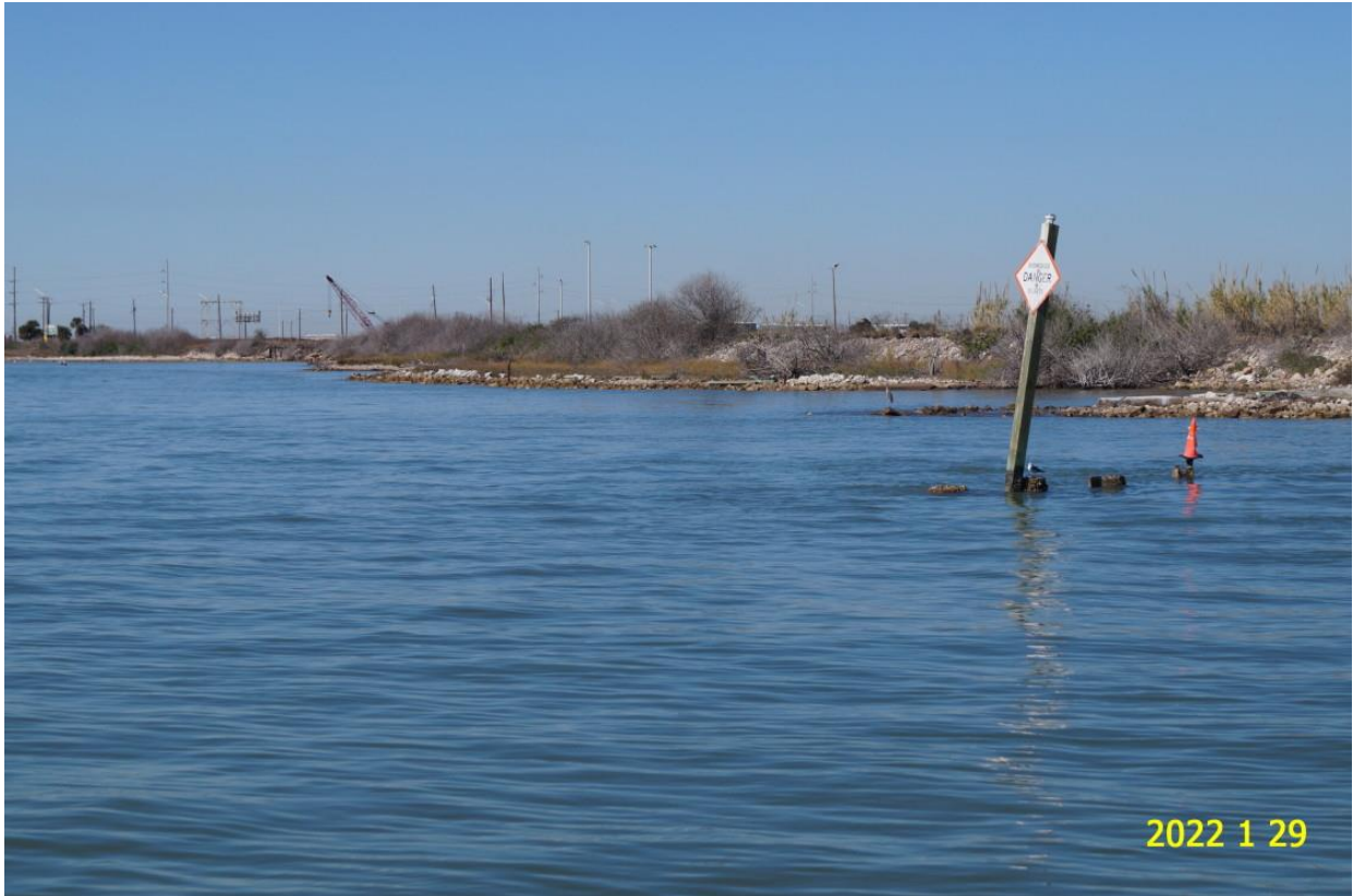
Point of Discharge just past warning sign, Harbor Island shoreline
