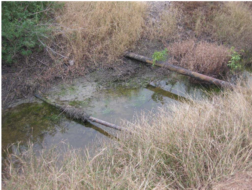
Photo 69 -Plot PL-19 drainage feature on southside of FM78.
