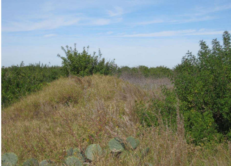
Photo 3 –Levee at southeast corner of HI looking northwesterly
