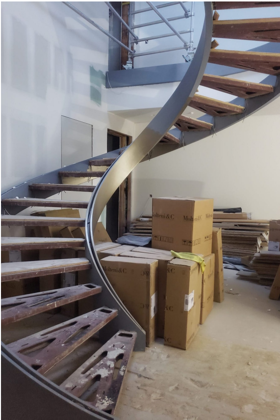
Curved staircase installation
