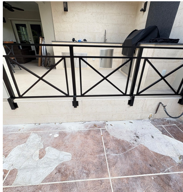
Clean panel spacing
