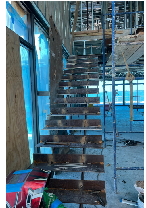
On-site stair installation
