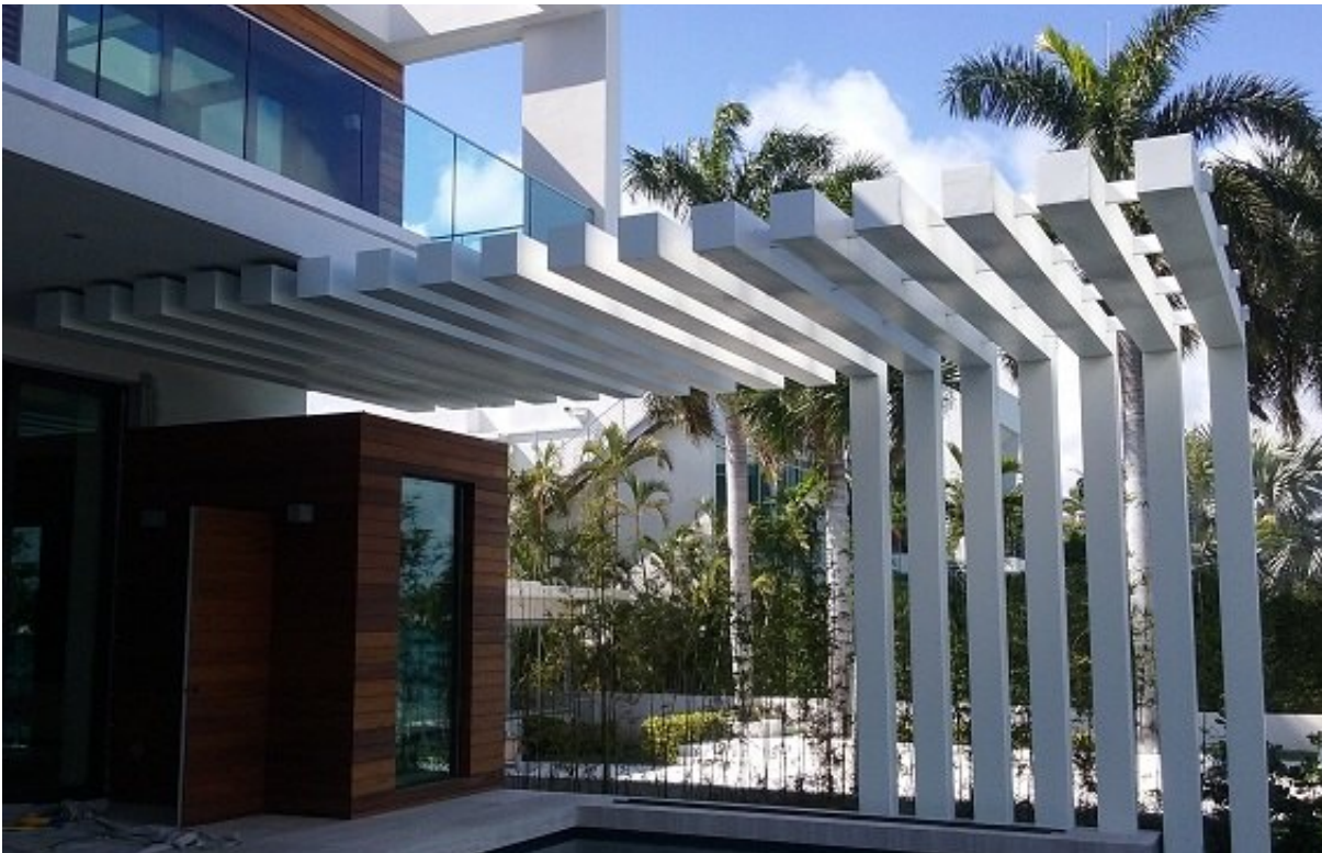
Aluminum pergola / exterior structure
