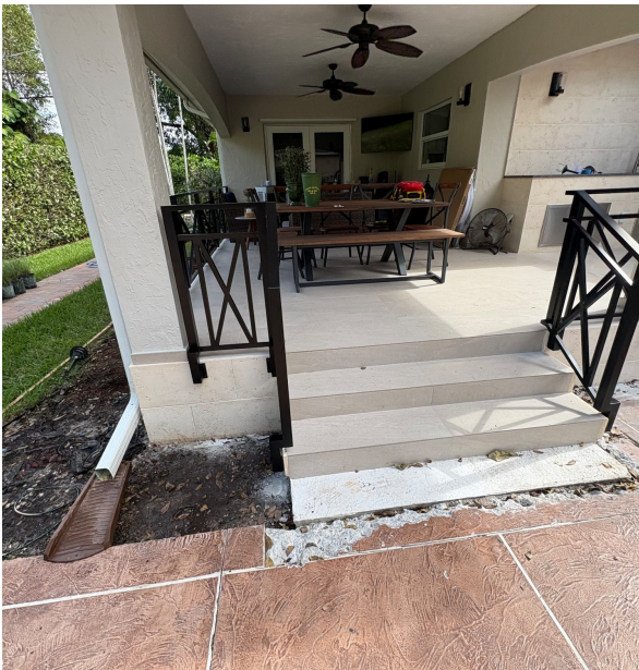
Entry stair railing
