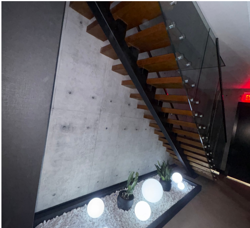
Steel, wood, and glass stair
