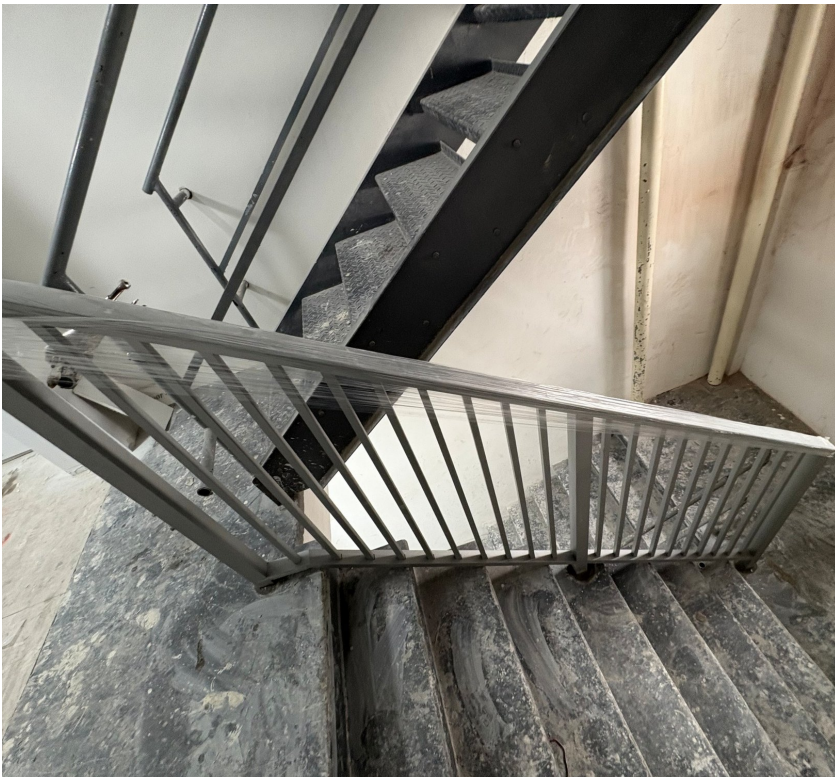
Interior stair railing
