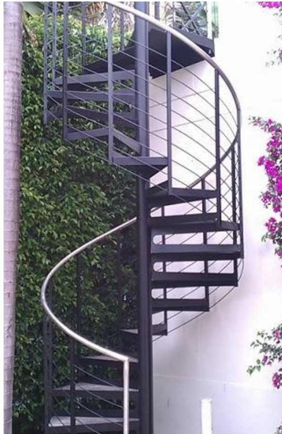
Spiral stair with custom rail
