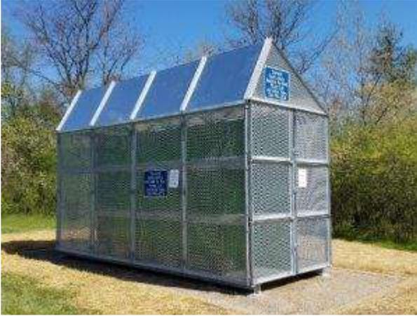
Boat lockers are now available along the Huron River in Ann Arbor. This prototype, designed and manufactured in Ann Arbor by Hosford & Company, can accommodate the majority of kayak and canoes. The lockers have six compartments that can fit up to two boats each. Each locker is modular so more lockers can be added as demand grows.
