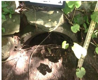
Clogged Structures with Sediment Buildup
