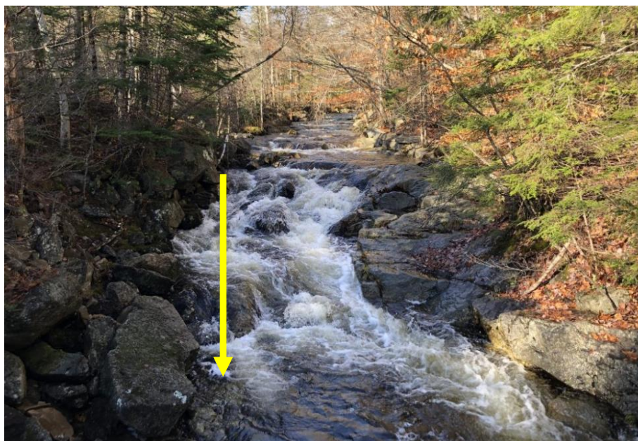
An example of a section of river upstream of the culvert inlet that has a sudden steep gradient.
