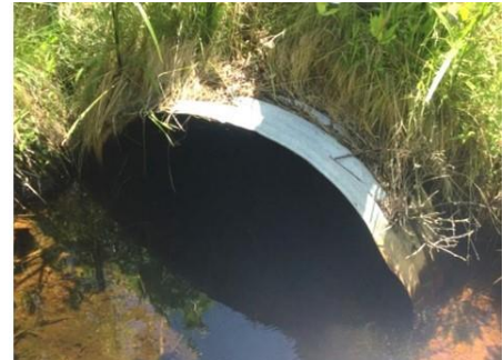
Clogged Structures with Sediment Buildup
