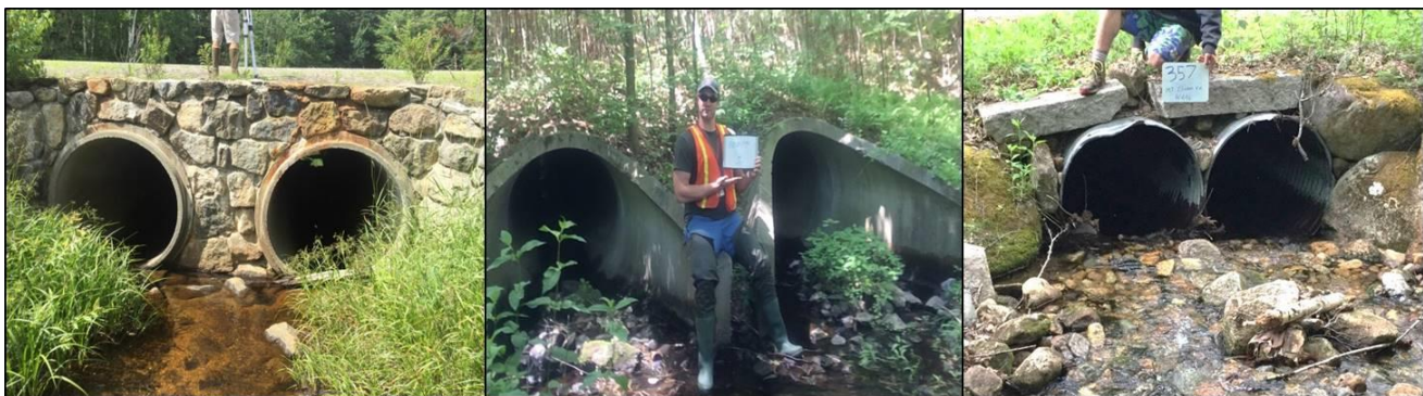
Identical structures at a crossing
