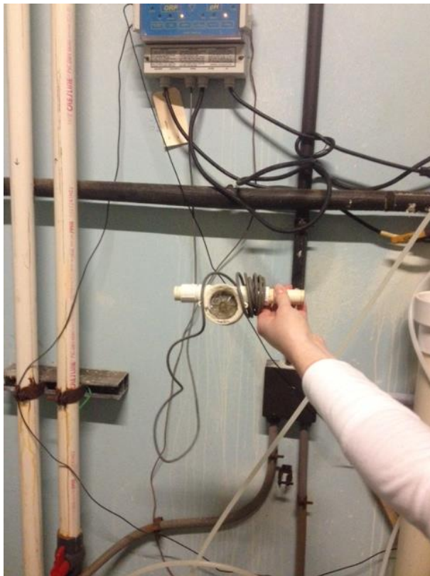
Broken Flow Switch (Not Acceptable)
