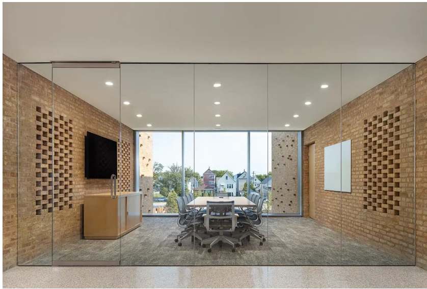
Structural masonry walls fronted with reclaimed Chicago brick define the offices within. Photo © James Florio
