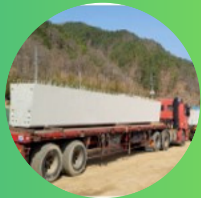
TRANSPORTING FLEX-C SEGMENT TO THE PROJECT SITE
