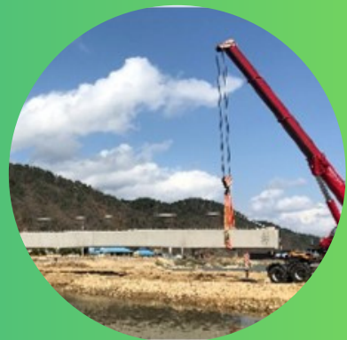
LAUNCHING THE FULLY ASSEMBLED AND STITCHED FLEX-C GIRDER.
