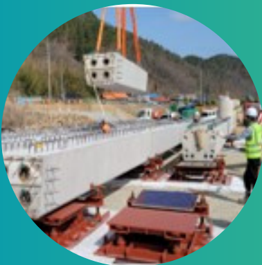
UNLOADING FLEX-C GIRDER SEGMENTS ONTO THE ASSEMBLY TABLE.
