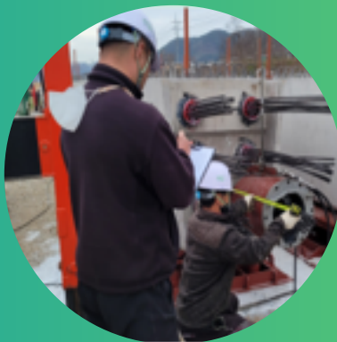
PERFORMING POST-TENSIONING TO STITCH FLEX-C GIRDER SEGMENTS.
