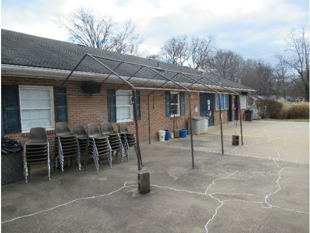
Shade structure frame overview
