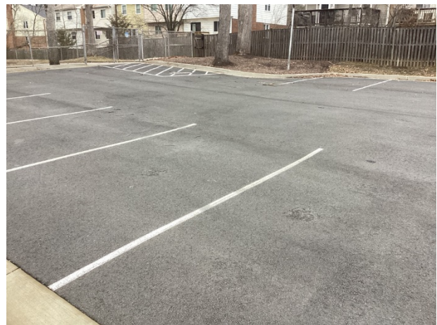
Asphalt pavement parking area overview
