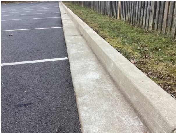
Concrete curb and gutter overview
