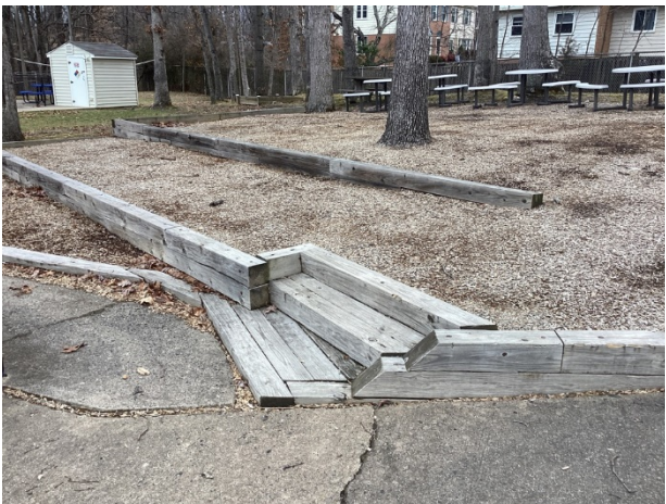
Timber retaining walls overview
