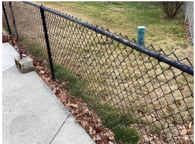
Safety chain link fence overview
