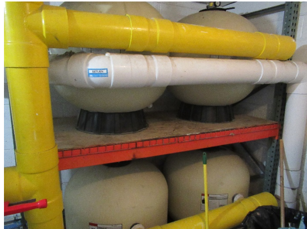
Main pool filters overview
