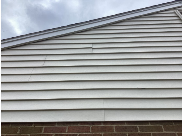
Vinyl siding overview
