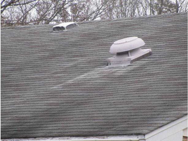
Asphalt shingle roof
