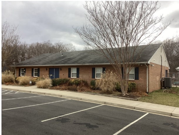
Community Center overview
