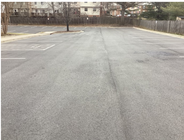
Asphalt pavement parking area overview
