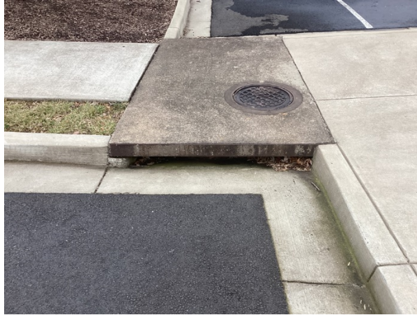
Catch basin overview
