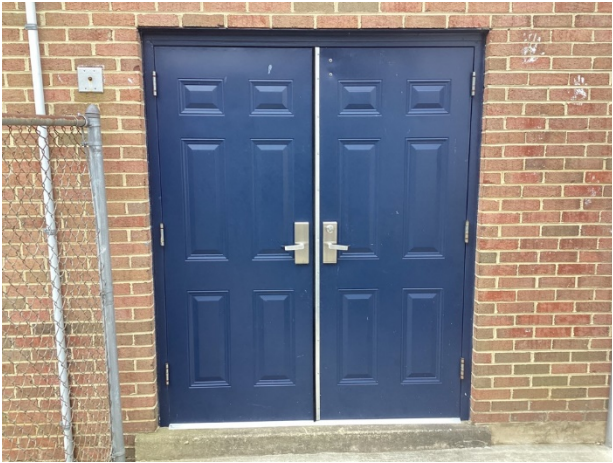
Side entrance doors overview
