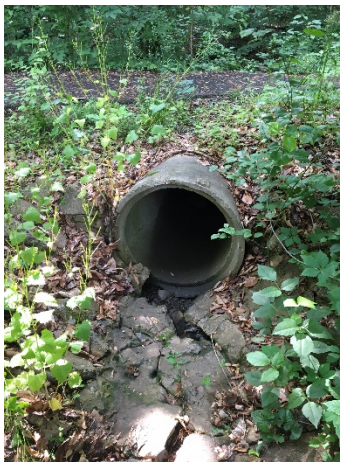
Pipe underneath trails
