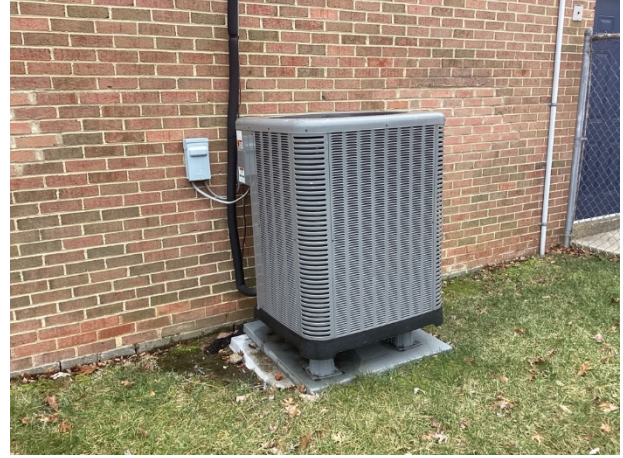
Condensing unit overview
