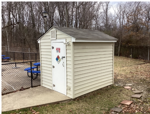
Wading pool shed overview
