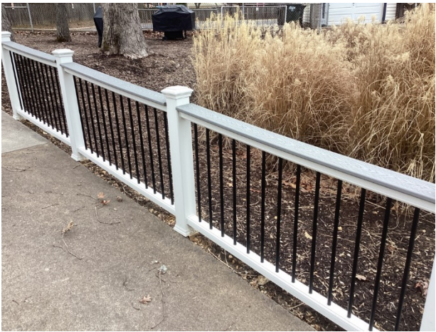
Vinyl fence overview
