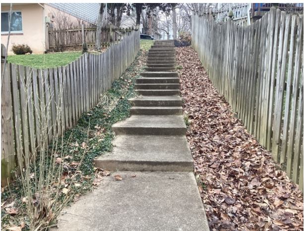
Concrete stairs overview, South trail, #2
