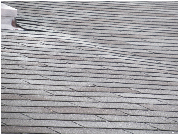
Asphalt shingle roof overview
