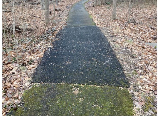
Asphalt pavement walking path repaired section
