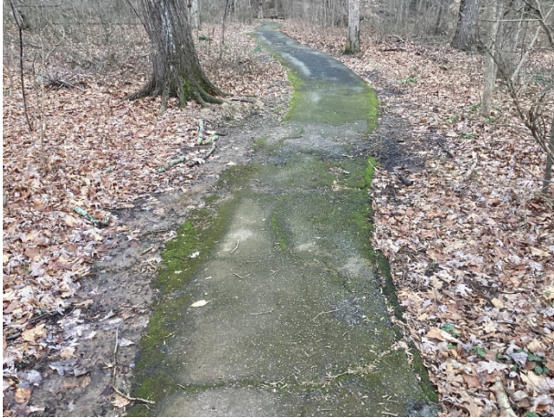
Asphalt pavement walking path overview
