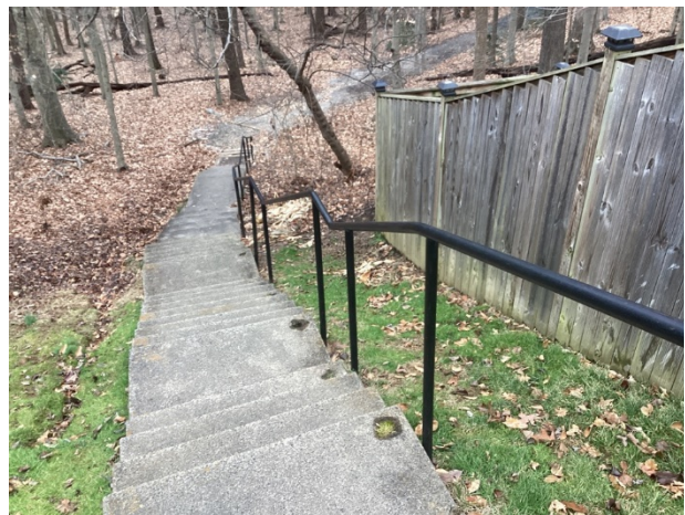
Concrete stairs overview, Steps leading from Ridge Ford Drive to Burke Station Park (Note: This staircase is the responsibility of Fairfax County Park Authority.)
