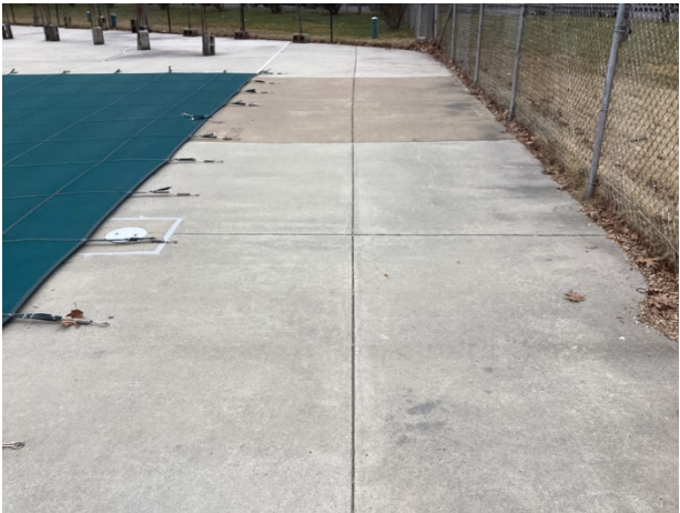
Concrete deck overview
