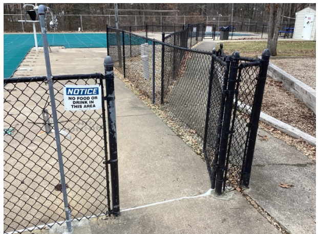
Main pool chain link gate
