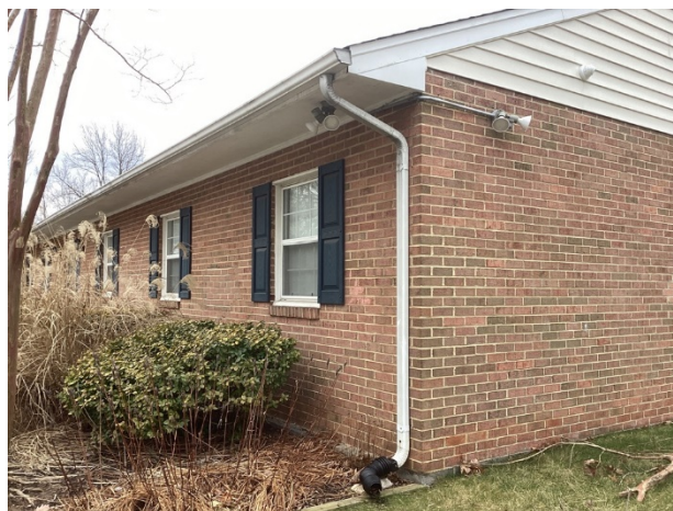
Gutter and downspout overview
