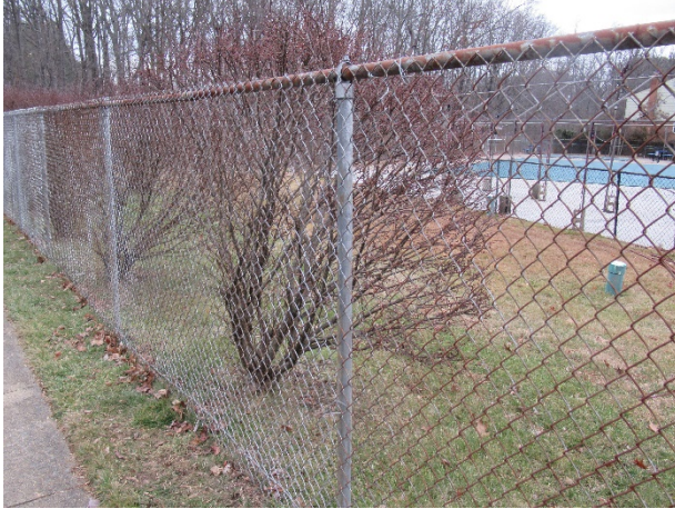
Security chain link fence overview
