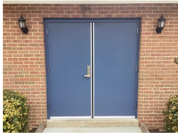
Main entrance doors overview
