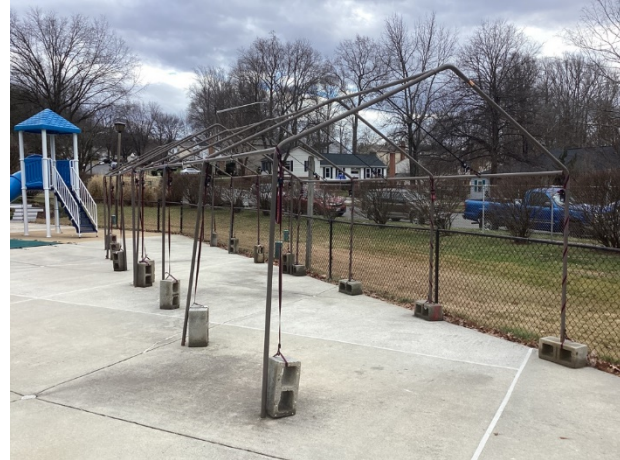
Shade structure frame overview
