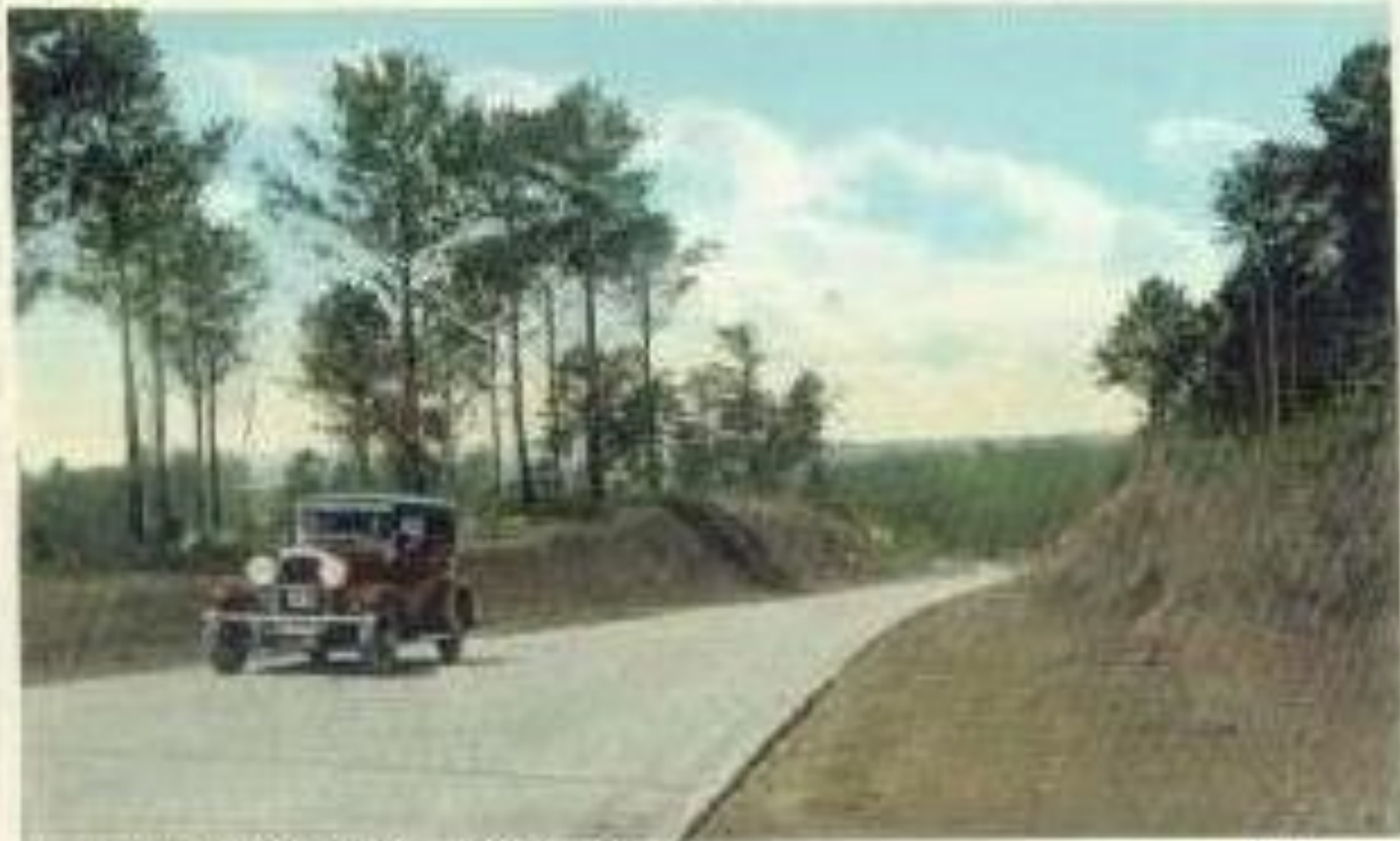
HIJWAY TO INDIAN SPRINGS, GA. STATE ROUTE 81
