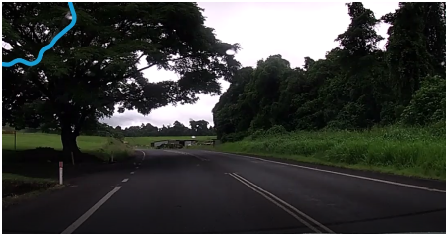
Figure B1 – Example of required pruning from overhanging tree branches, located on Palmerston Highway, 13.7 km from Bruce Highway
