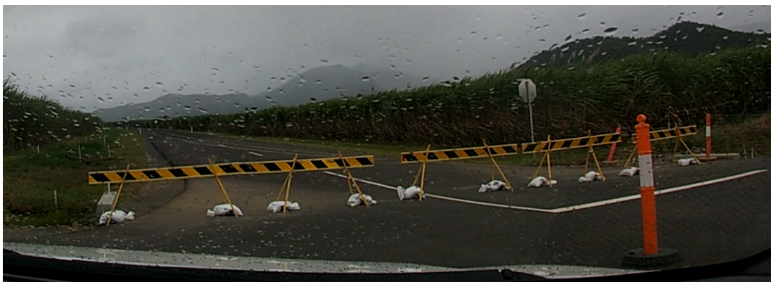
Figure 9 – Recently constructed Warner-Harris Connector Road (photo taken 26 th May 2021 on Harris Road)
