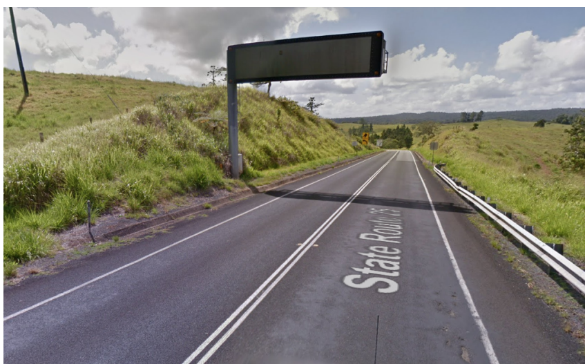
Figure B3 – Overhead Electrical Road Sign
