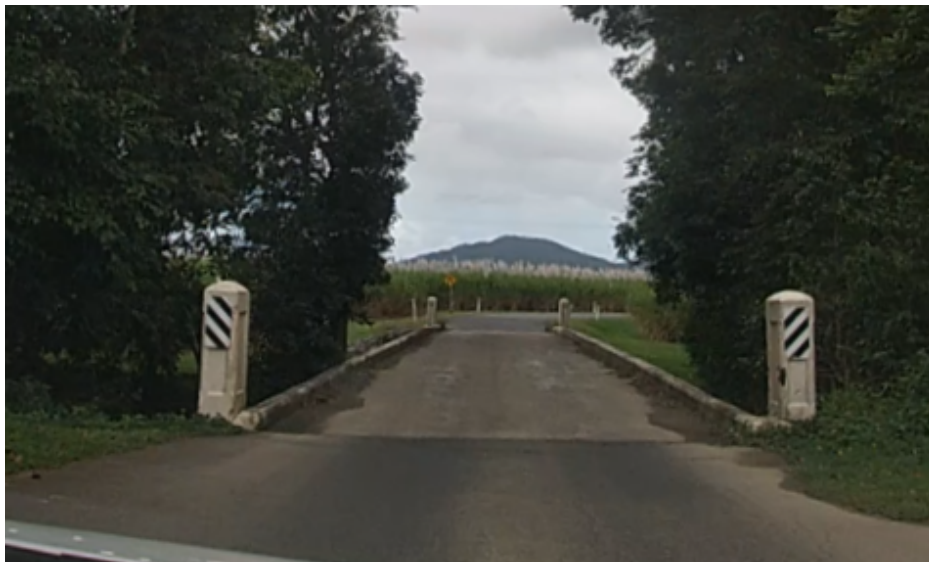
Figure 10 – Culvert Bridge on Page Road (photo taken 26 th May 2021)
