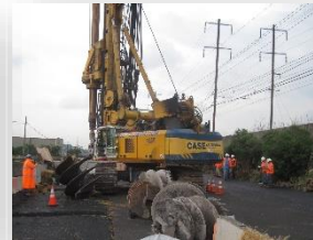
Portal Bridge Capacity Enhancement: "Shaft and Piling" testing
