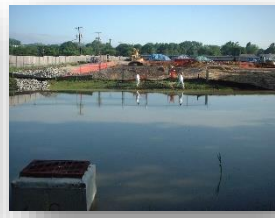
Sediment control basin constructed as part of soil remediation project
