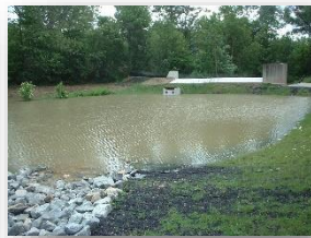
Sediment control basin constructed as part of soil remediation project
