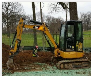
Pesticide remediation in wooded area by source removal and blending
