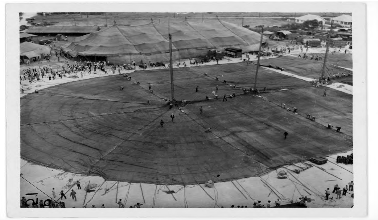
Lacing it all together. The Big Top was constructed in sections which included middle and end pieces that were laced together on the show lot. Hobson’s logs referred to these sections as “Ends” and “M.P.” (below).
