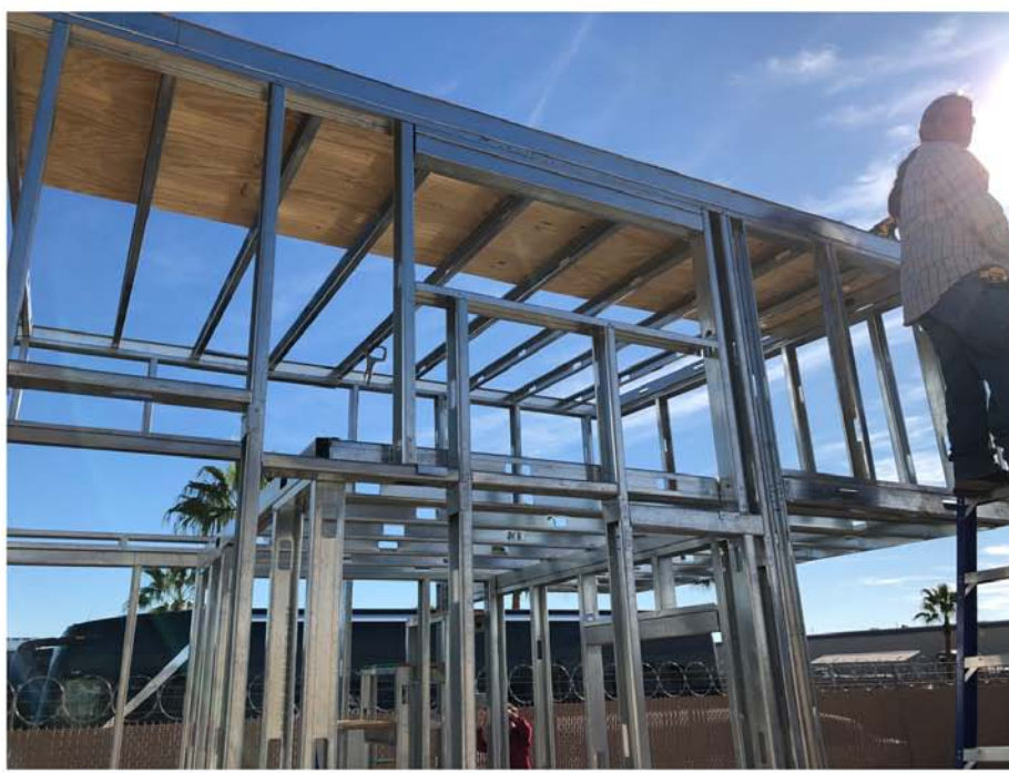
ThinHaus Frame with Roof Trusses and Sheathing
