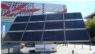
Ground Mount Solar Panels
