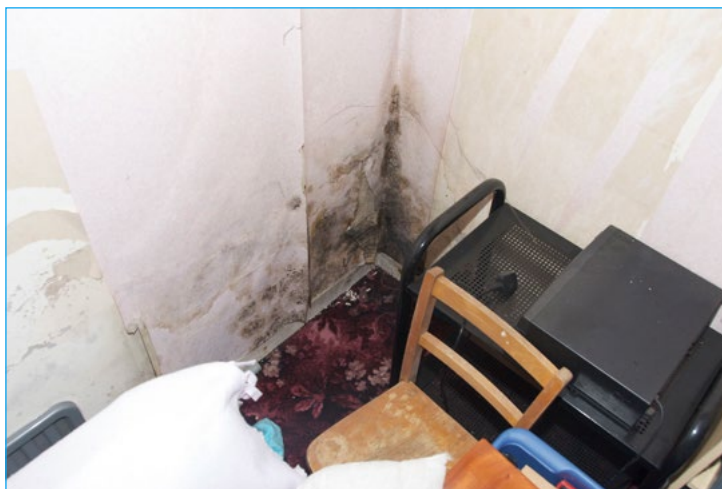
Figure 12: Mould growth and dampness.
