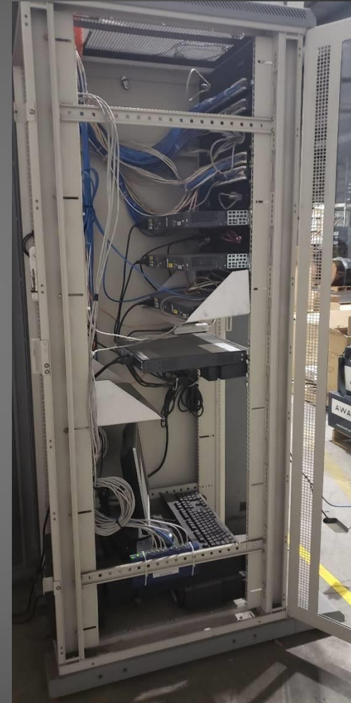
All switch's got cleaned up & wires organized in IT cabinet
