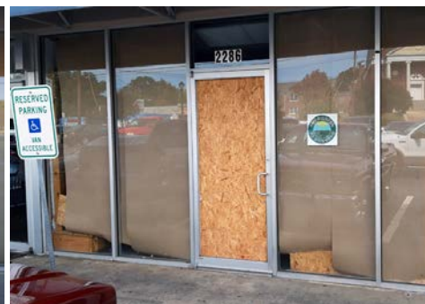
The buildout begins for our first CBD retail Store
