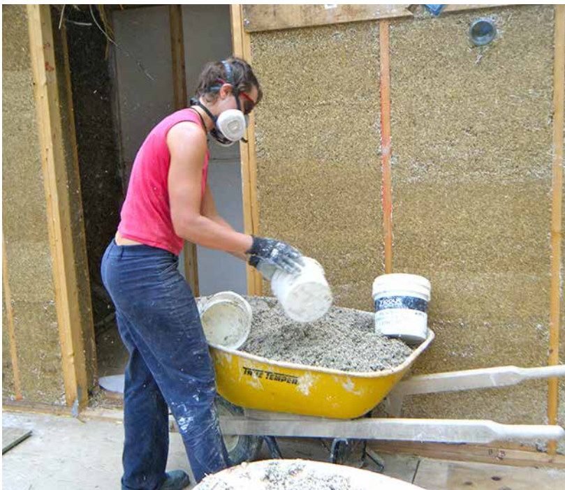
Shovels work well for placing hempcrete up to a comfortable height, and then small buckets become more practical.
