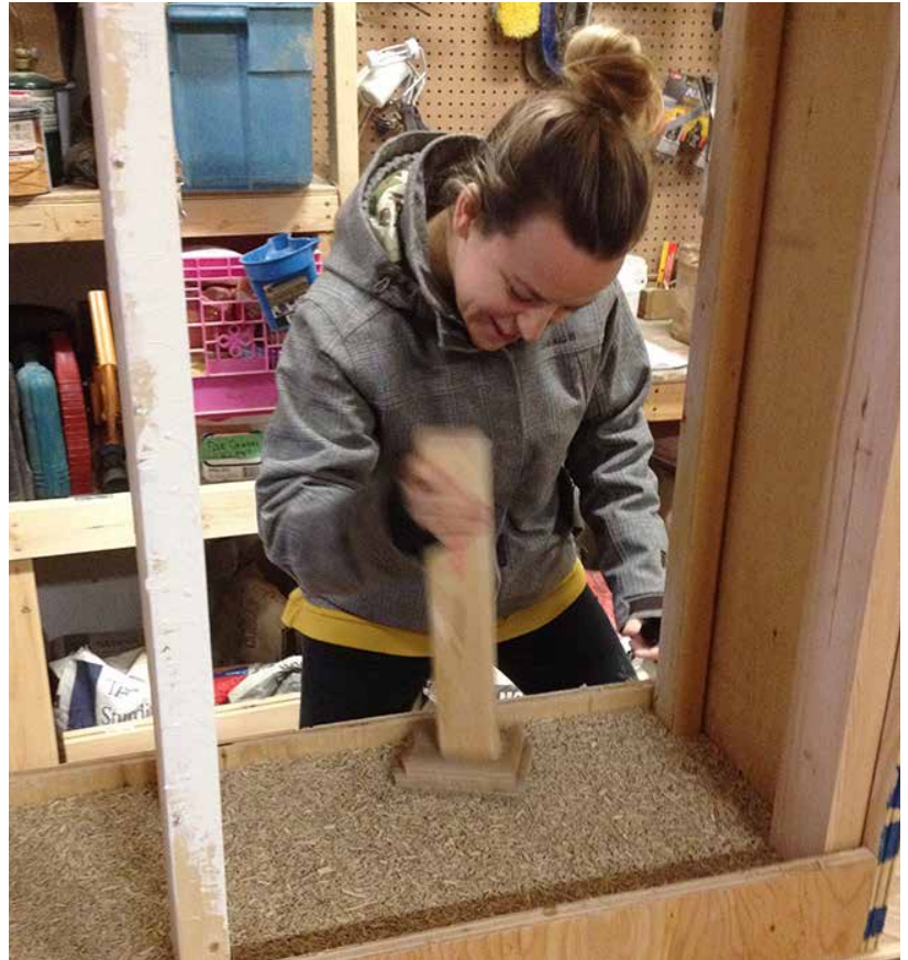
A tamping stick with a relatively wide contact area can prevent applying excessive pressure. A gloved hand may be the best option for pressing hempcrete into forms.
