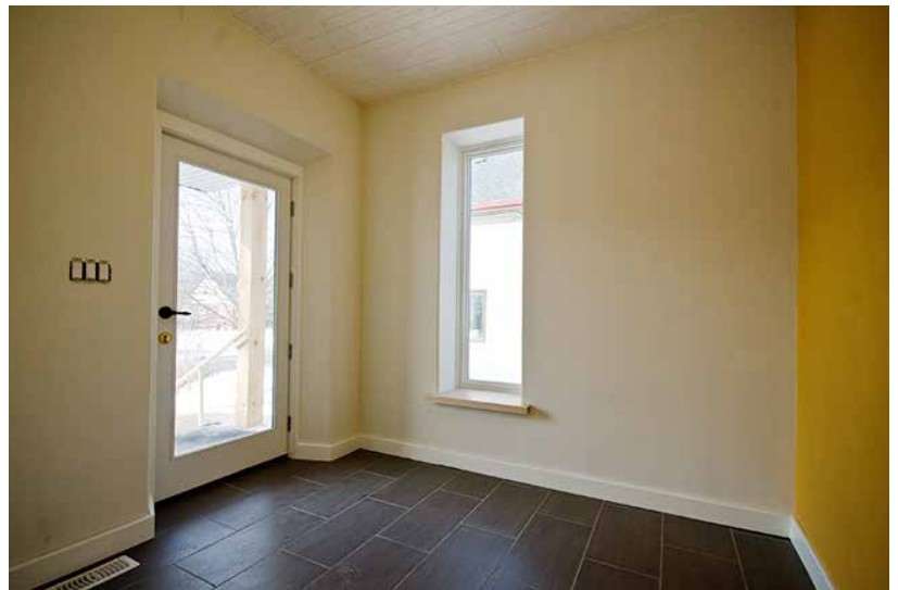
Conventional drywall can be applied over unconventional natural fiber insulation. In this case, the final finish is lime paint, which helps maintain the look and feel of natural materials.
