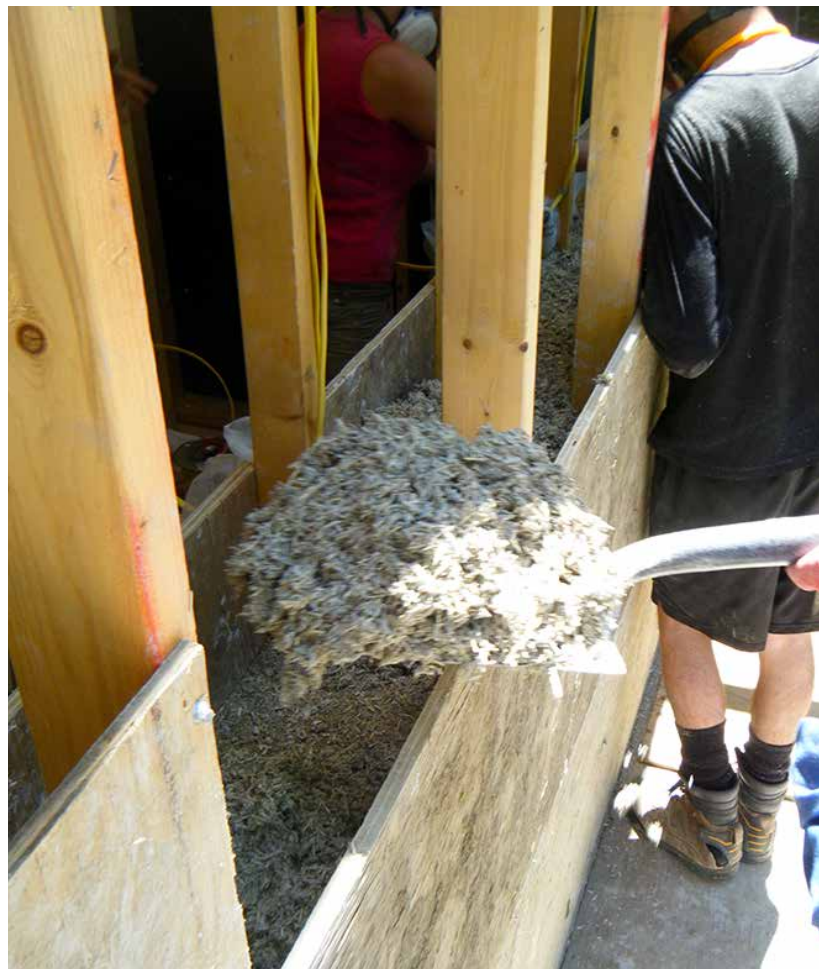
Hempcrete is loose and crumbly until tamped.
