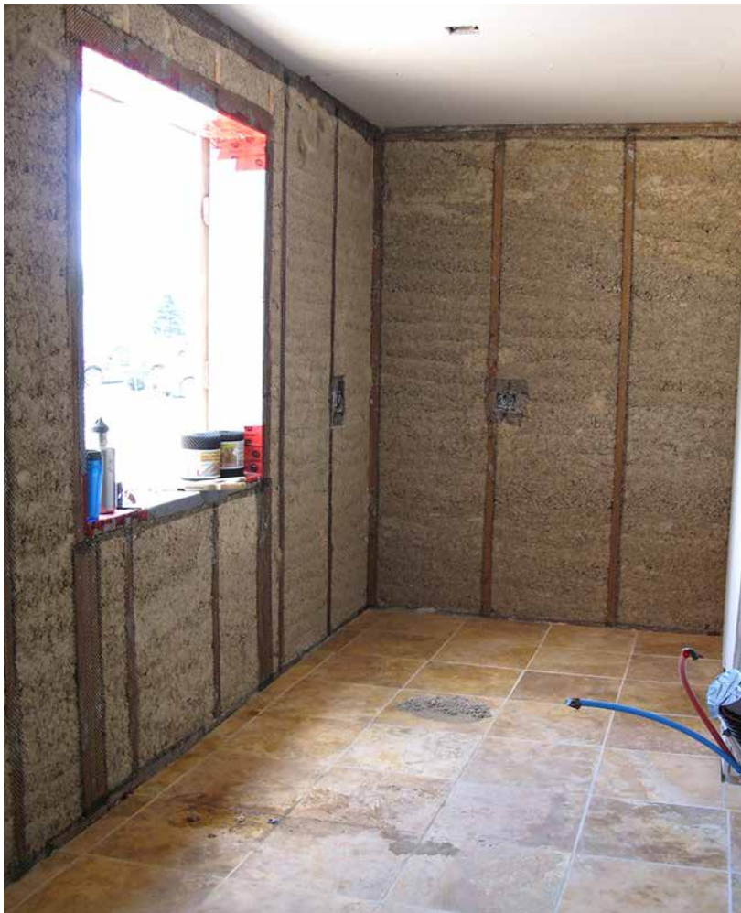
A finished hempcrete wall is satisfying to look at!
