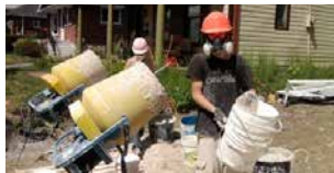
This crew is properly attired for mixing hempcrete, but they won't get viable hempcrete out of this kind of barrel-style concrete mixer.
