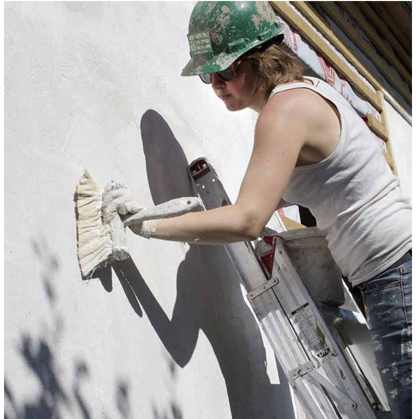
A lime wash adds color and protection to an exterior lime plaster.
