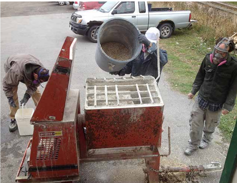
Typical horizontal shaft mortar mixers do an adequate job of mixing hempcrete, and are widely available in a range of sizes.
