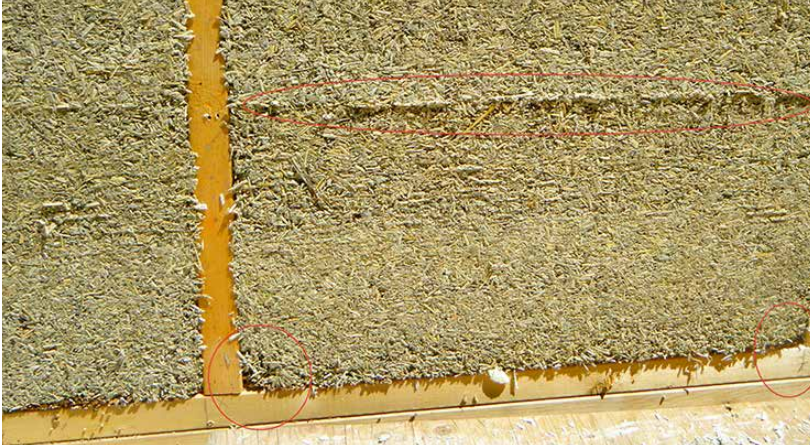
As soon as the wall is finished, inspect for voids and fill them with fresh mix.
