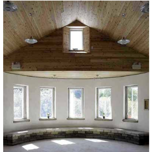
Hempcrete trim can easily be formed to any shape, and makes attractive exterior trim. On the interior, hempcrete can be trim and windowsill material (and bench top as well).
