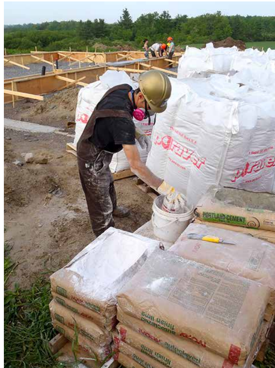
Metakaolin (Metapor from Poraver, in this case) and other pozzolans often come in Super Sacs rather than individual bags. Cost and ease of use are often better in this larger format.
