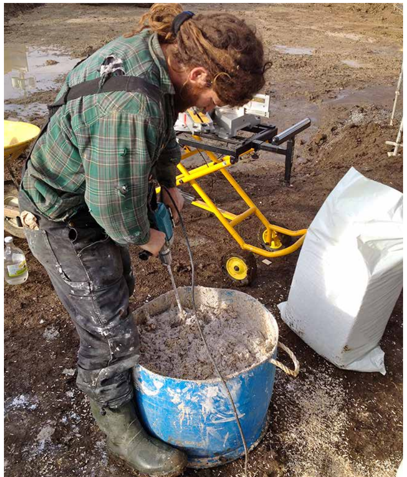
Specialty vertical shaft mixers are very good at mixing hempcrete, but may be harder to source than horizontal shaft versions.
