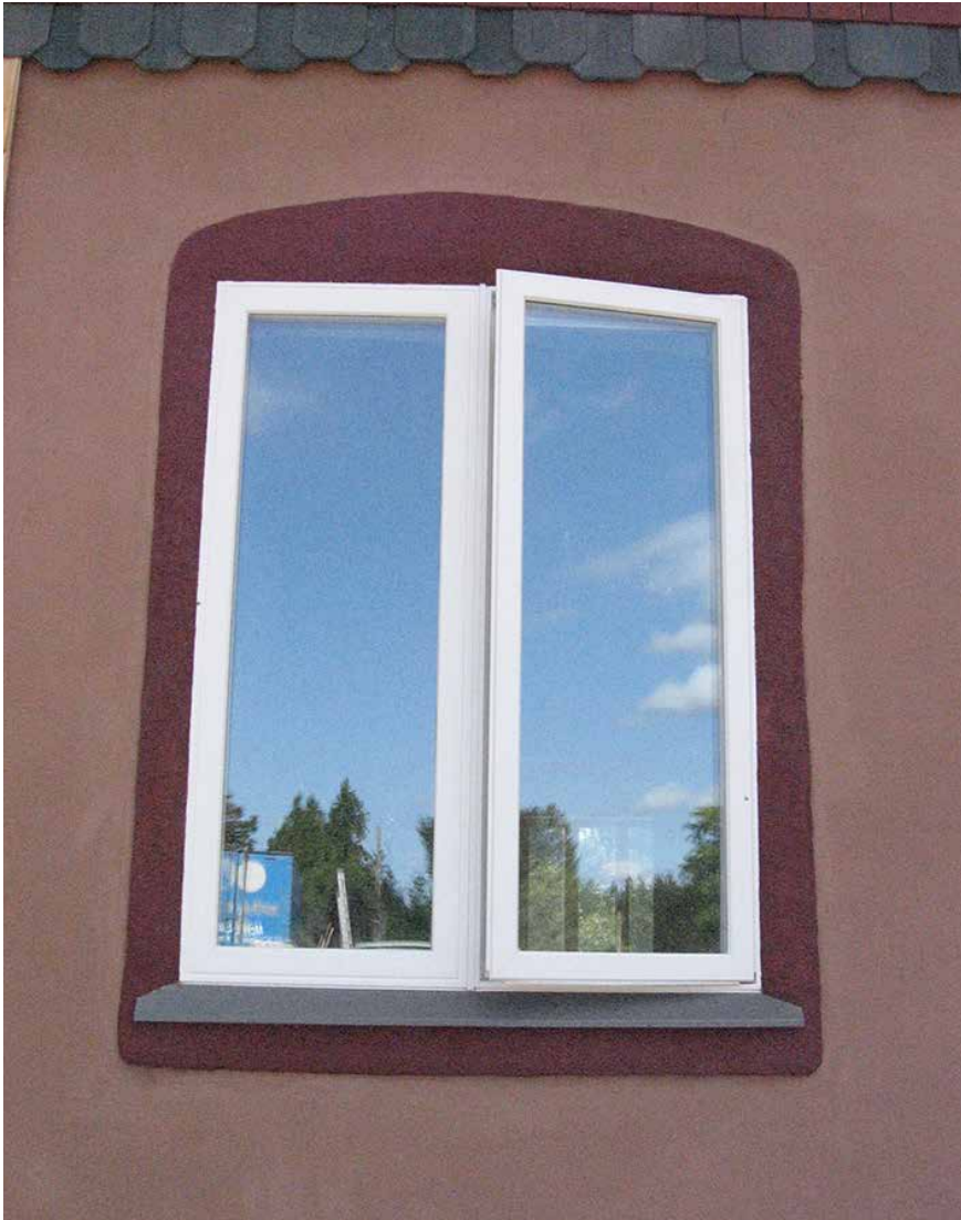
Hempcrete trim can easily be formed to any shape, and makes attractive exterior trim. On the interior, hempcrete can be trim and windowsill material (and bench top as well).
