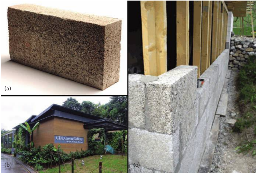
FIGURE 7.31 Hemp–lime blocks (made with a mixture of woody hemp core [hurds], lime binders, and water) in building construction. (a) Hemp–lime block. Photo by Scott Lewis (CC BY 2.0). (b) A building in the Philippines with walls constructed of prefabricated hemp–lime blocks (public domain photo). (c) Hemp–lime blocks utilized as insulation on the exterior of standard wood-frame construction. Photo by Olivier DuPort (CC BY 3.0).
