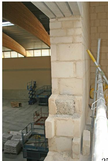
FIGURE 4.7: Hempcrete blocks filled with lime hemp concrete [81]
