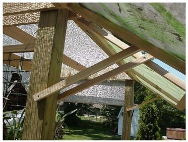
Since the stand sits on concrete pavers and the uprights are pressure-treated, I have not experienced any signs of rot on the wood in seven years. I am careful to
