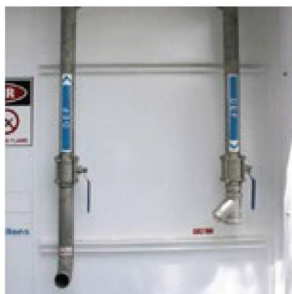
On-loading and off loading connection pipes.
